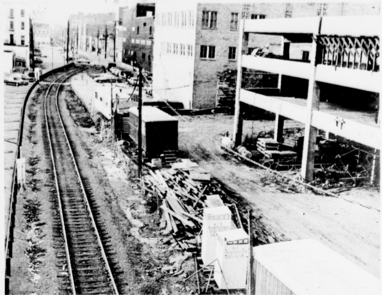
As part of Lexington's Railway Plan, this track will be removed soon from the downtown area. Such action further emphasizes increase use of automobile and the decline of railway passenger
