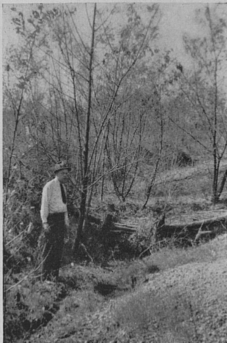
Black locust trees planted the Spring of 1934 which have, with the aid of check dams, about reclaimed this once badly gullied area.
