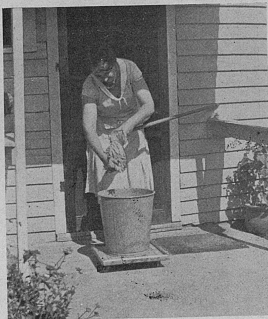
The "kitchen chariot" is a labor-saving device that is becoming popular. It is a board on rollers on which to move a wash bucket about the floor.
