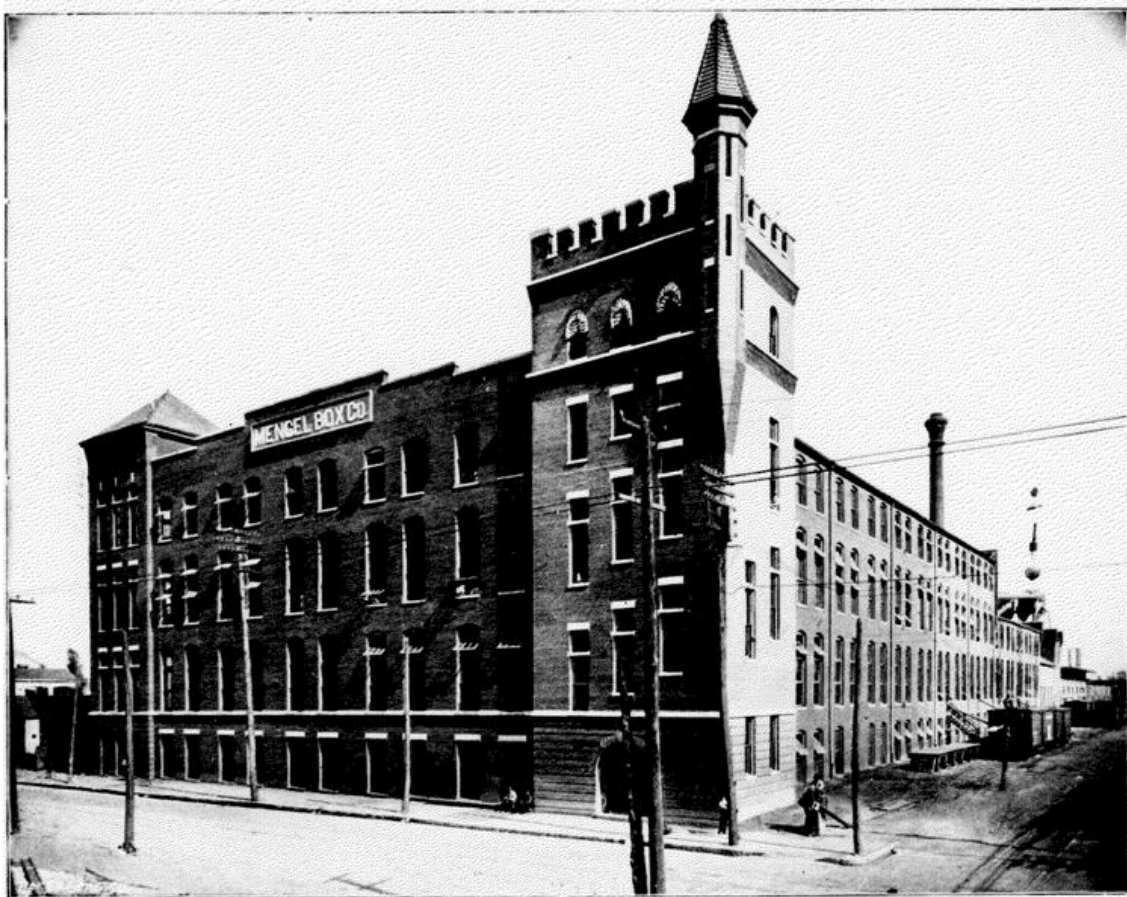
156 ft. x 500 ft. Factory at Louisville, Ky.
