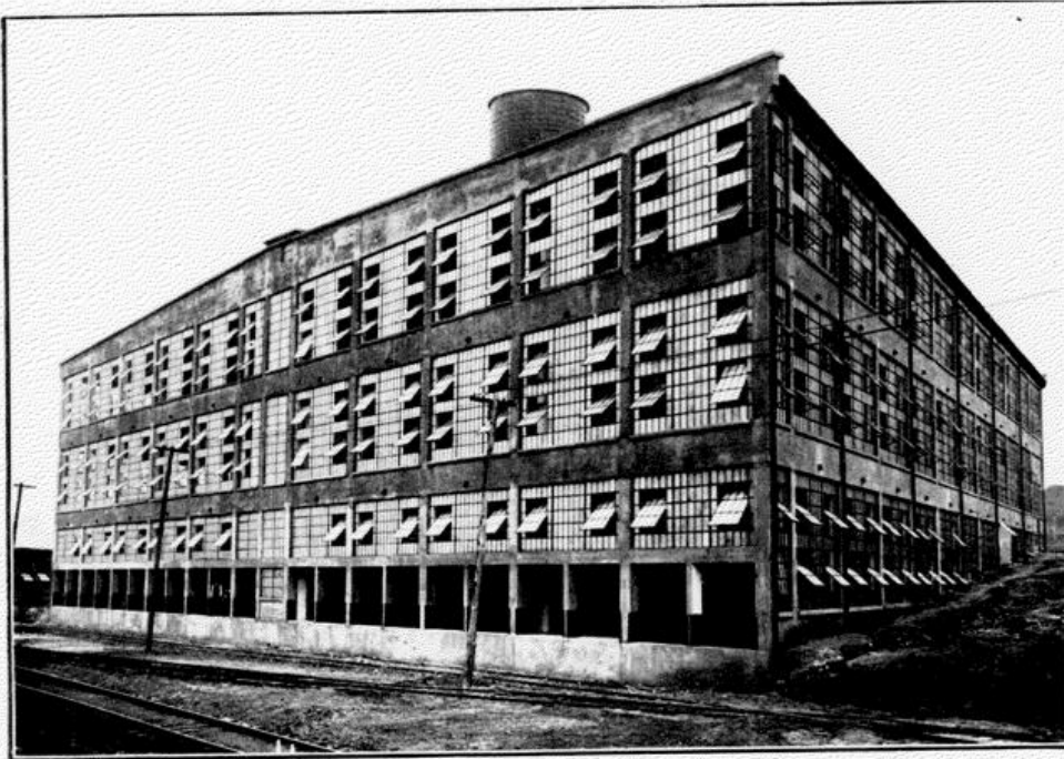
180 ft. x 200 ft. Factory at Winston-Salem, N. C. Reinforced Concrete
