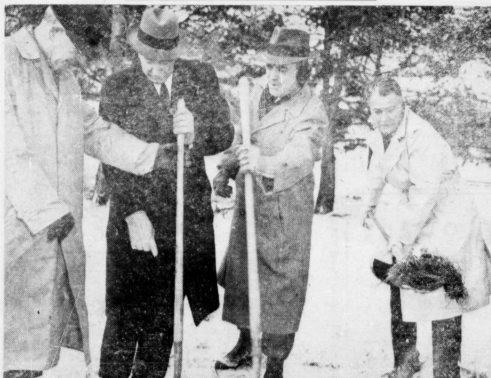
Spindletop Ground Breaking
