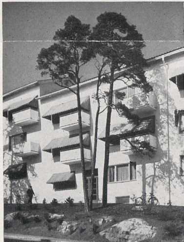
Stockholm: Cooperative apartments built on land rented from the city on a 60-year lease.
