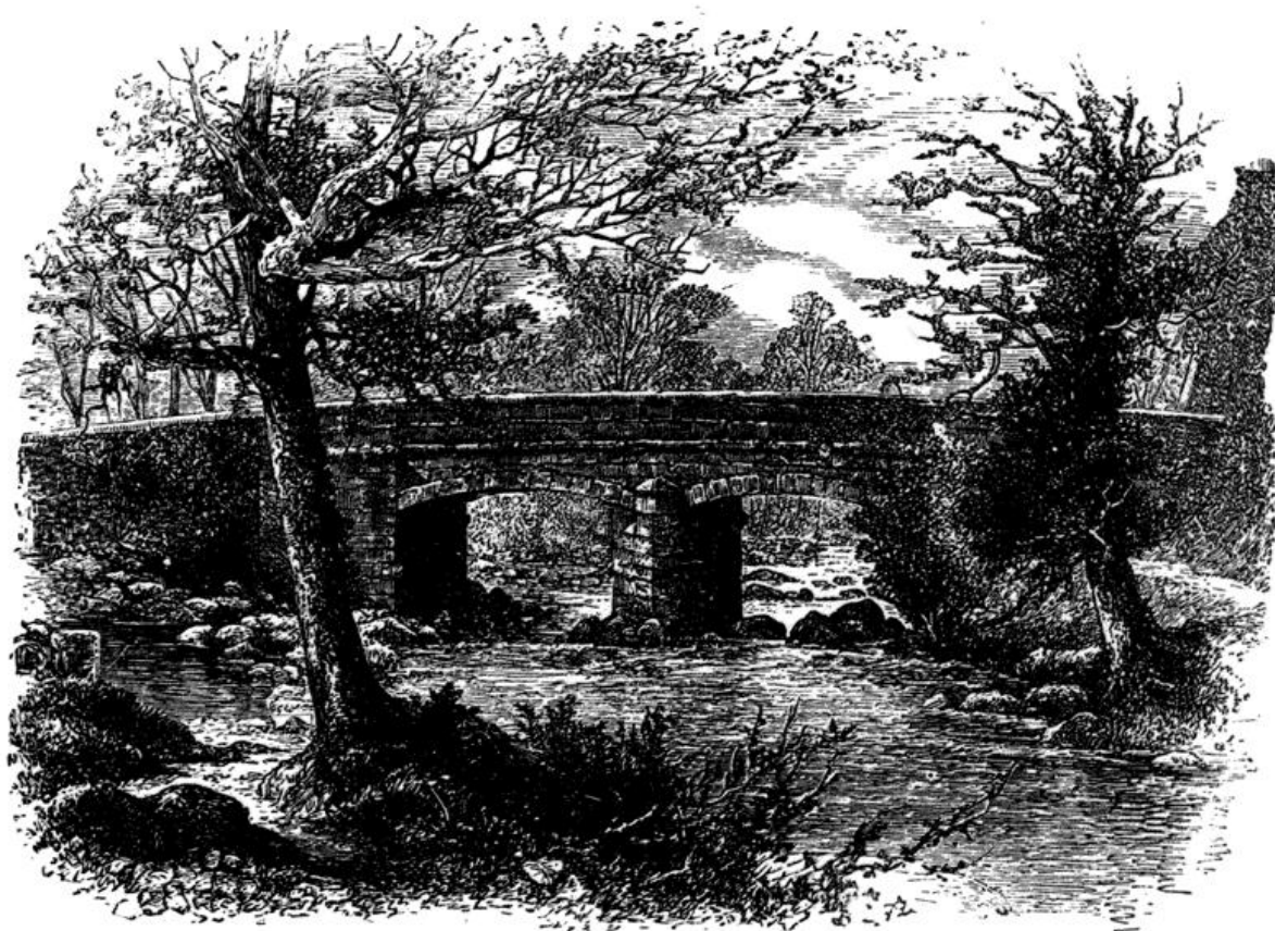
BRIDGE OVER THE PLYM (PLYMOUTH).
