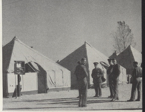
Training camps today are far better equipped than they were in 1918. Thanks in many cases to the WPA, they have proper drainage and sewerage, and either ample barracks or tents with concrete foundations and electric lights—like these at Fort Hancock, New Jersey.
