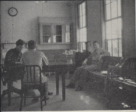
Army posts , to accommodate a prospective land force of 1,400,000 men, will need more and better facilities. The WPA has already done work at 80 percent of all Army reservations. This is the receiving room of a WPA-built infirmary at Fort Moultrie in South Carolina.
