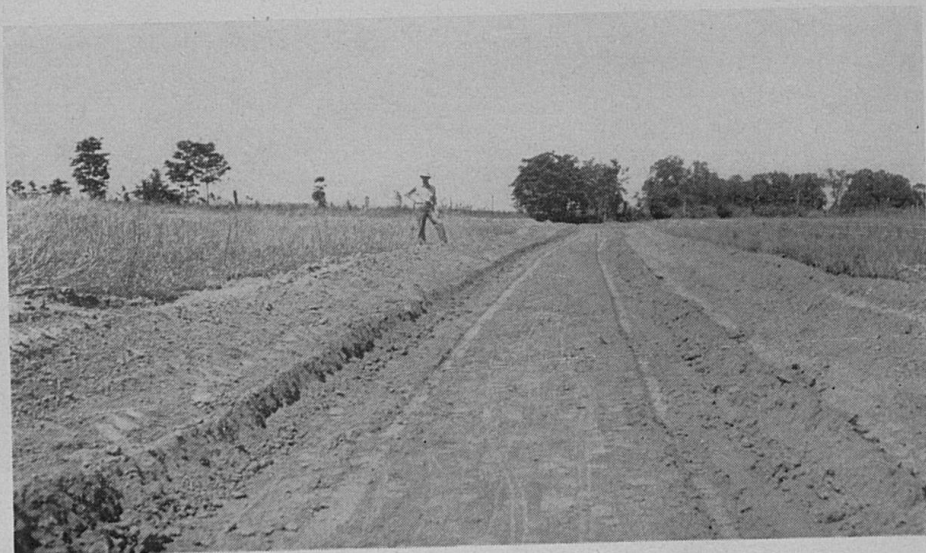
Fig. 6. An outlet channel cut to proper depth and width with terracer grader.
