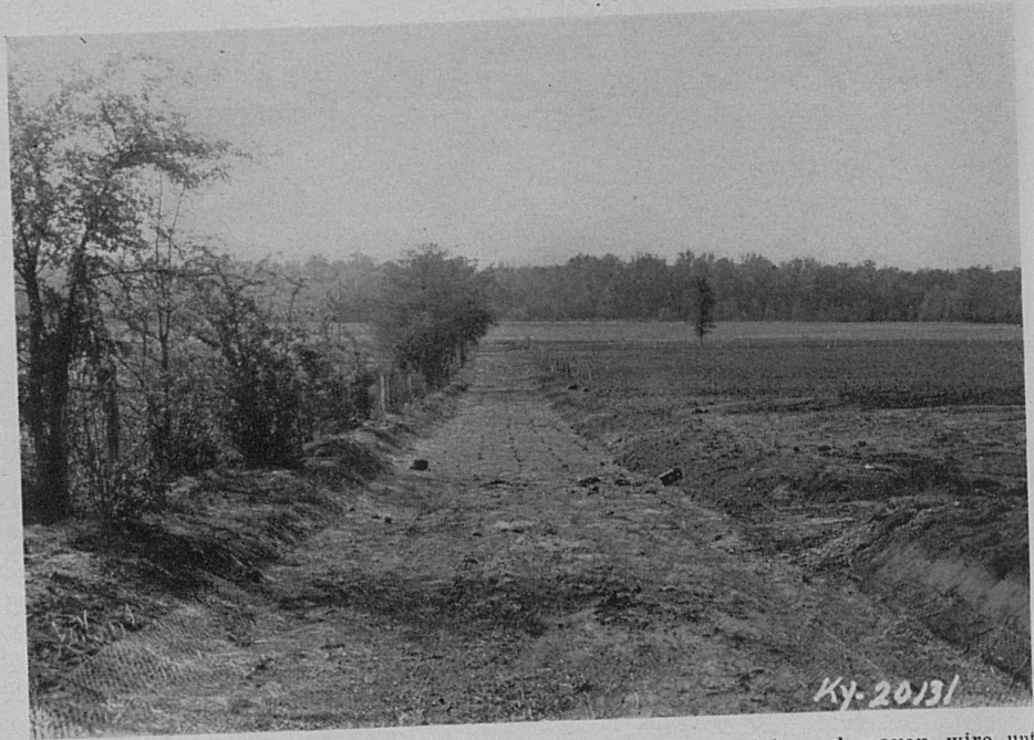
Fig. 8. An outlet protected from erosion by a straw mulch and woven wire until vegetation is established. (Courtesy of Soil Conservation Service.)
