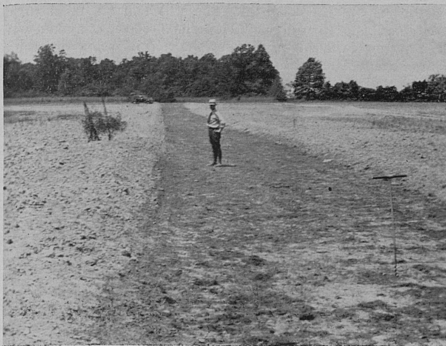
Fig. 4. A well-graded outlet channel.
