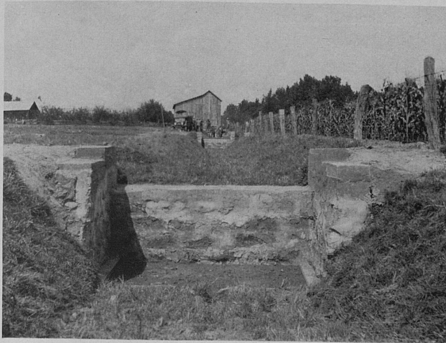
Fig. 31. Rubble masonry dam for a terrace outlet.
