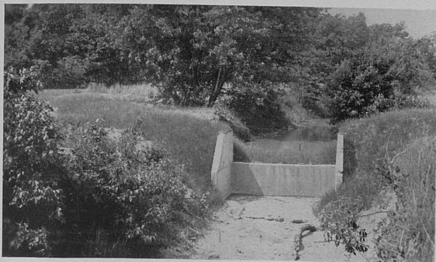
Fig. 33. Typical small concrete dam in gully.
