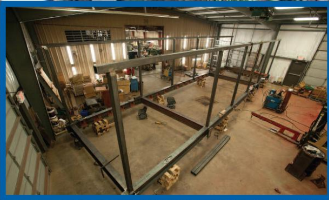
House construction begins on campus.
