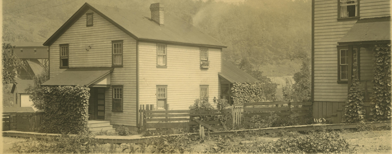
Typical Miner's House
