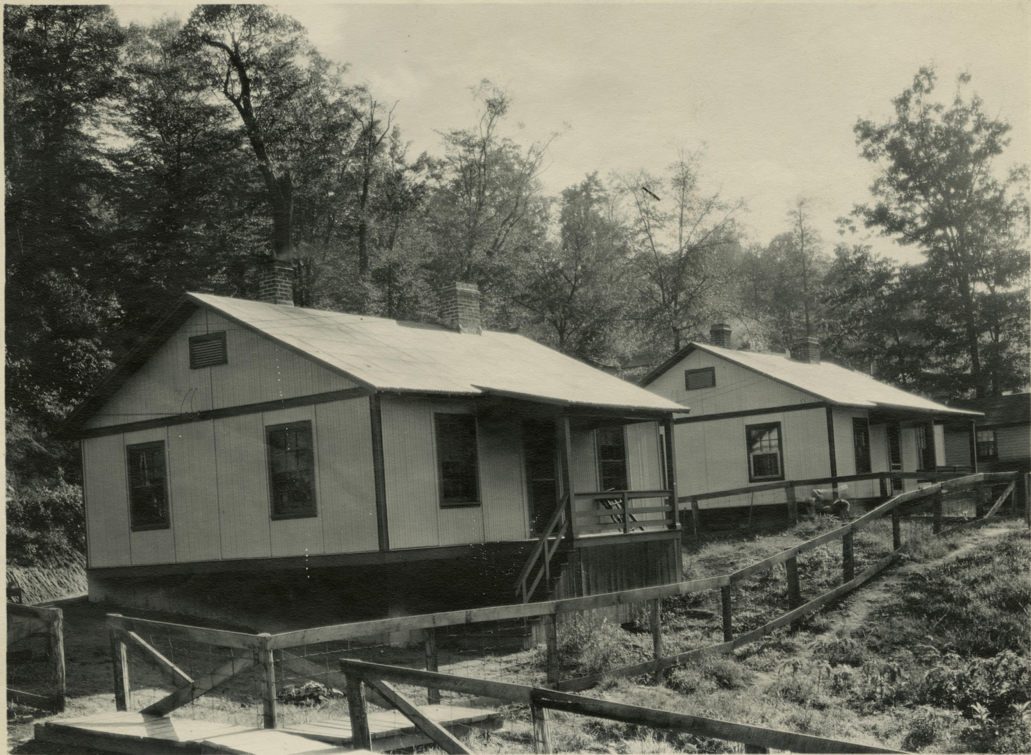
2242 New portable houses at Jenkins. 1908-11.
