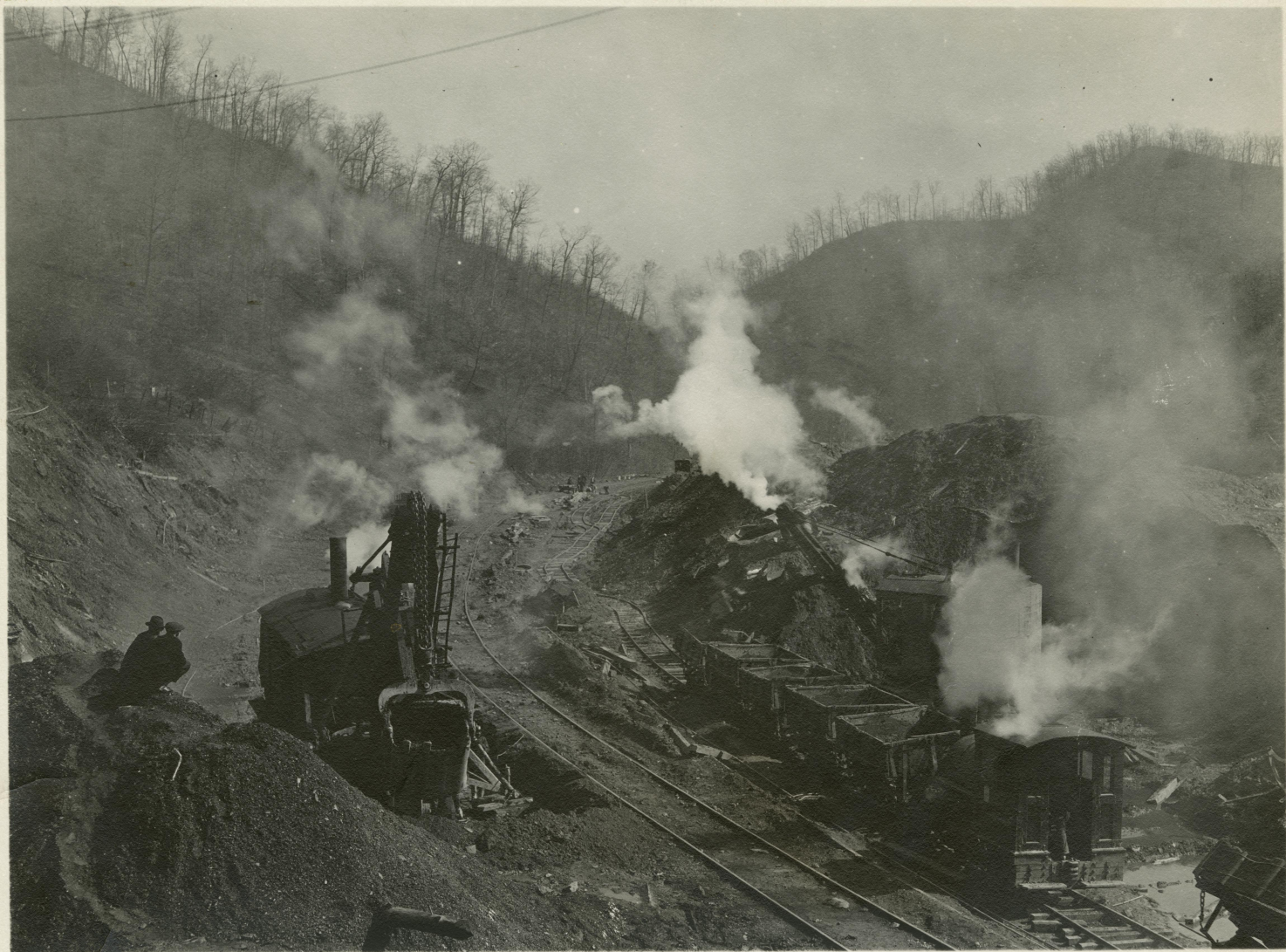
2341 - 201 Slide - Small shovel loading dinky cars. 3-6-23.
