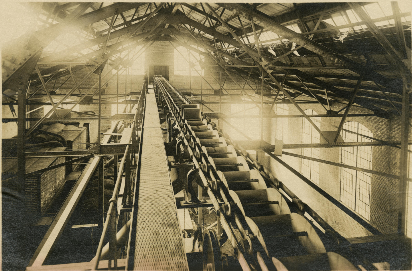
Conveyor in Power Plant
