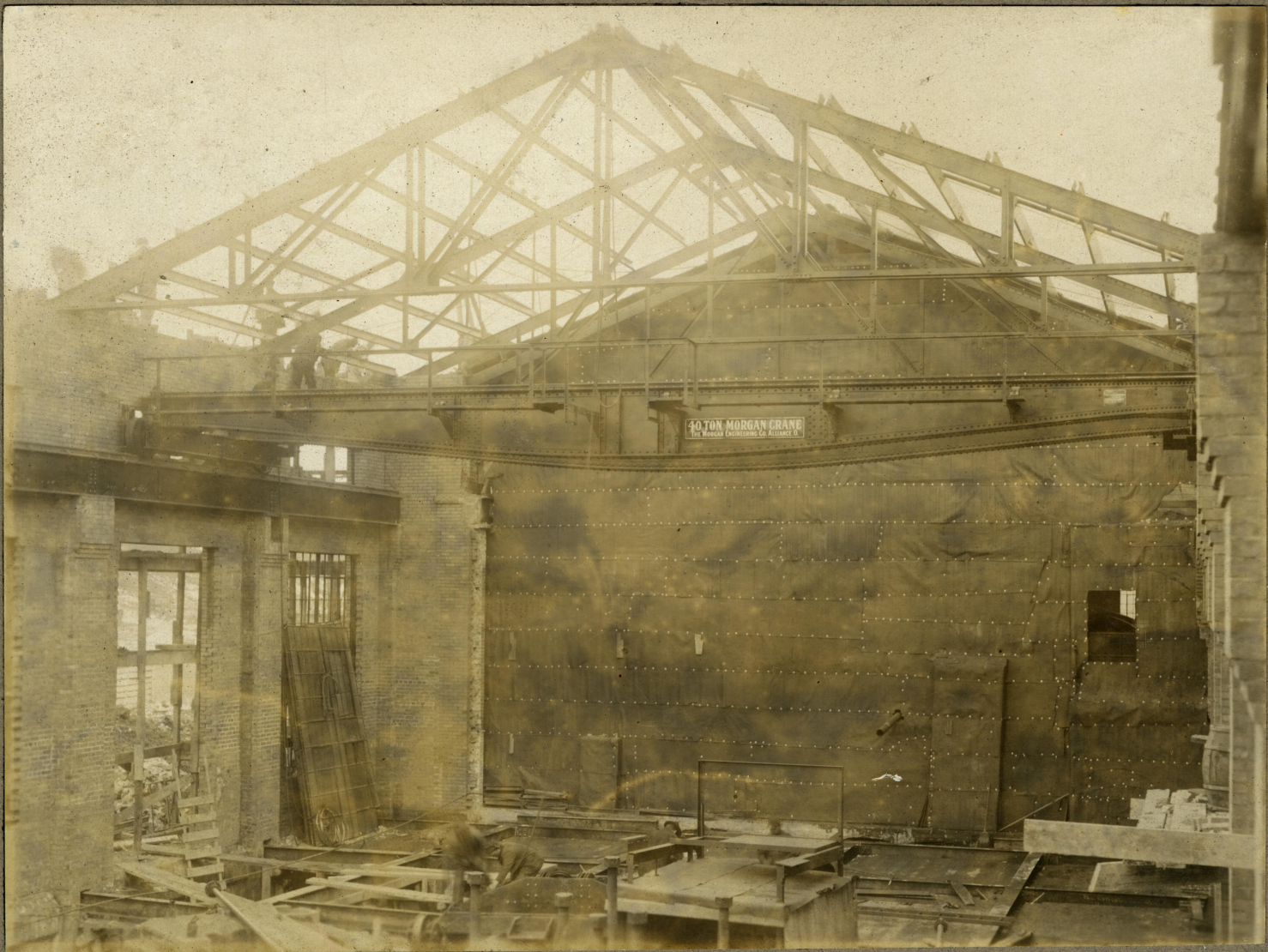
40-Ton Crane ~ Dec. 23, 1914
