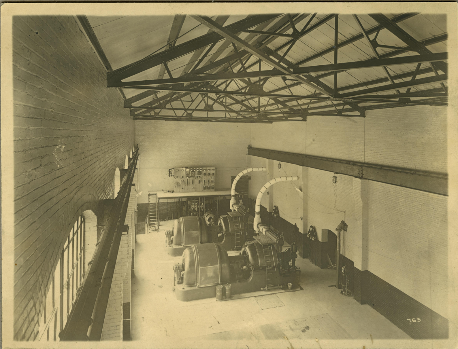
Central Power Plant- Turbine Room
