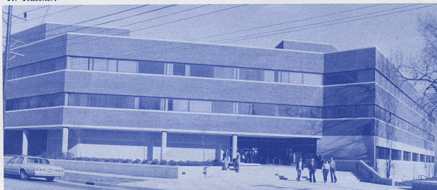
Mining and Mineral Resources Building — Rose Street and Clifton Avenue
