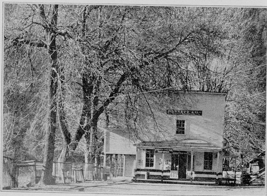
FIGURE 12.— THE BULLION BUYER IS PAYMASTER TO THE SMALL-SCALE PLACER MINER Bullion buyers perform an important economic function in the small-scale gold-mining industry. They are usually storekeepers who, operating in the vicinity of the creeks, buy gold as a side line to their merchandise business. A general store of the type at which gold is bought is shown in the lower view; the upper view shows the sale of a small quantity in process.
