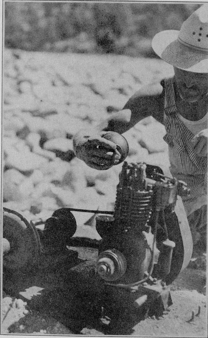
FIGURE 13.— A LIGHTWEIGHT ENGINE-AND-PUMP OUTFIT
