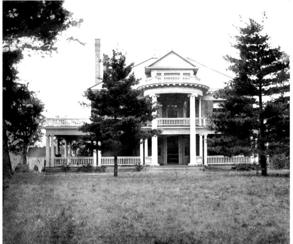
Front Elevation of Residence.
