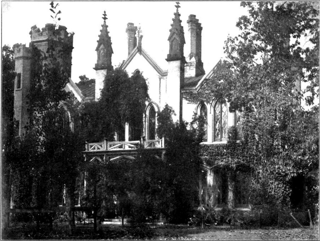
Front Elevation of Residence.
