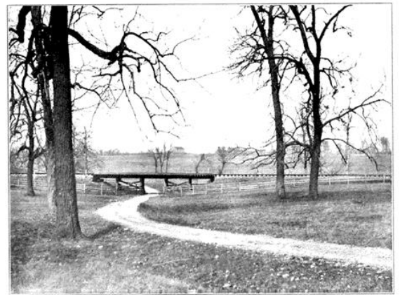
Where the Driveway Goes Under the Bridge.
