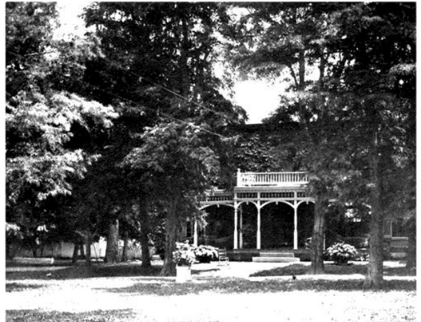
General View of "The Maples."
