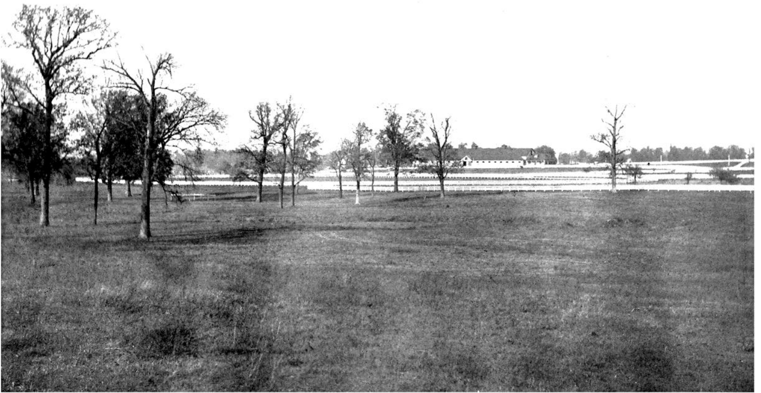
BIRDSEYE VIEW OF SENORITA FARM ON IRONWORKS ROAD, SHOWING PADDOCKS AND BARNS IN THE DISTANCE.
