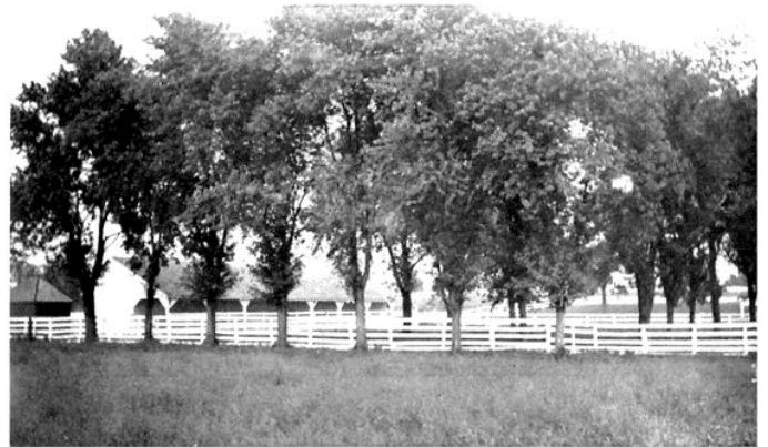
Locust Grove Which Shelters Some of the Buildings.
