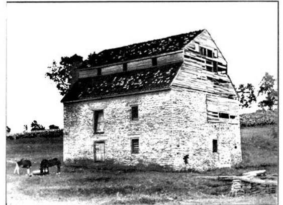
The Century-Old Mill at South Elkhorn.
