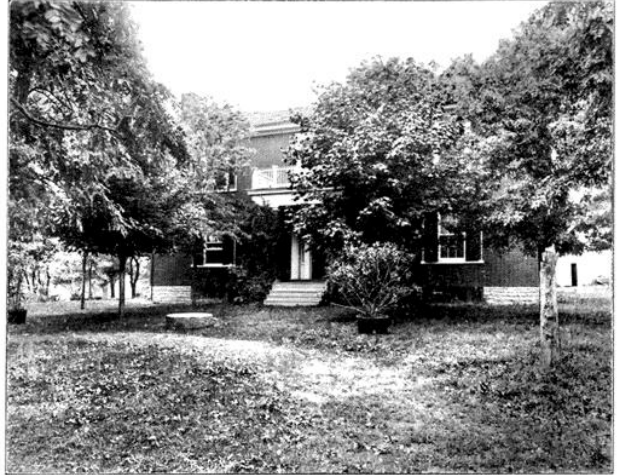
Cottage at Locust Heights.
