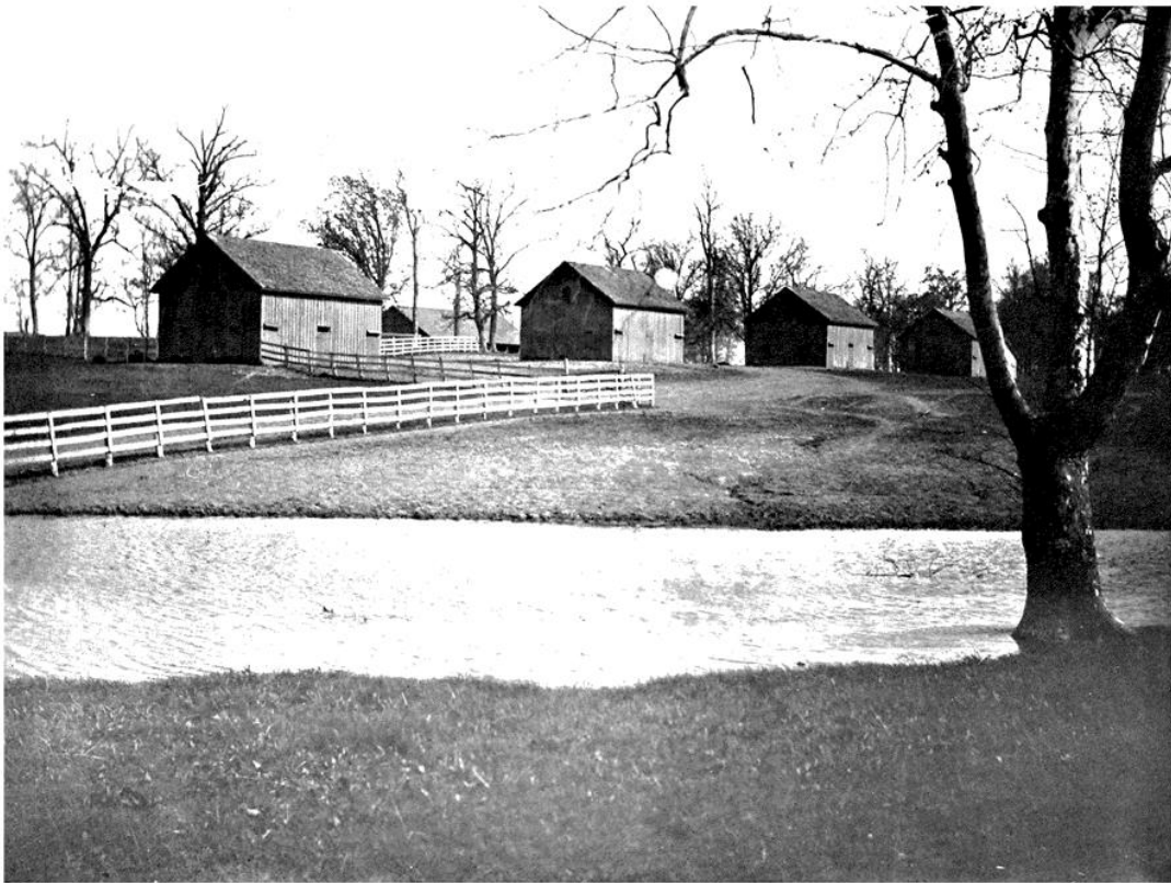
Several of the Barns, With Pond in Foreground.
