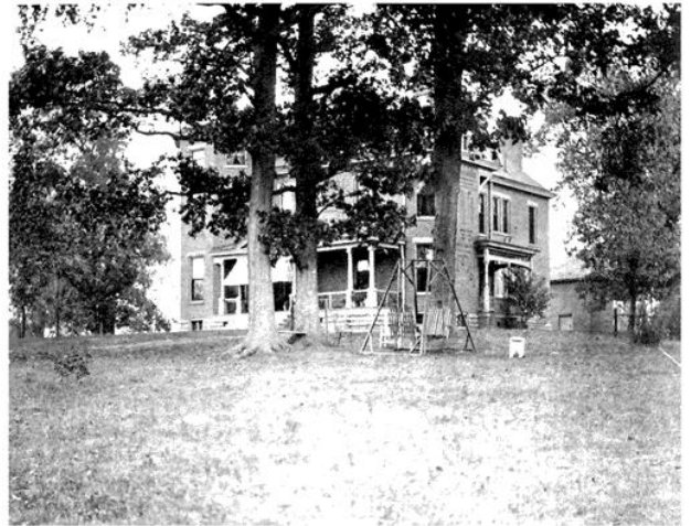
View of Residence from the Driveway.
