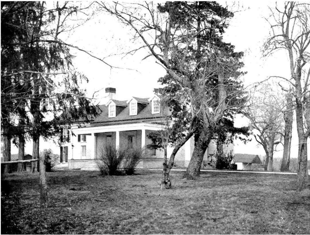
View of House Through Trees.
