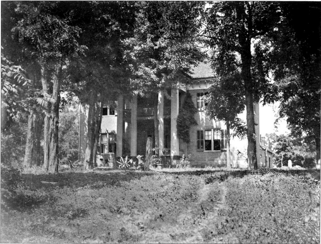
Front Elevation of Residence.
