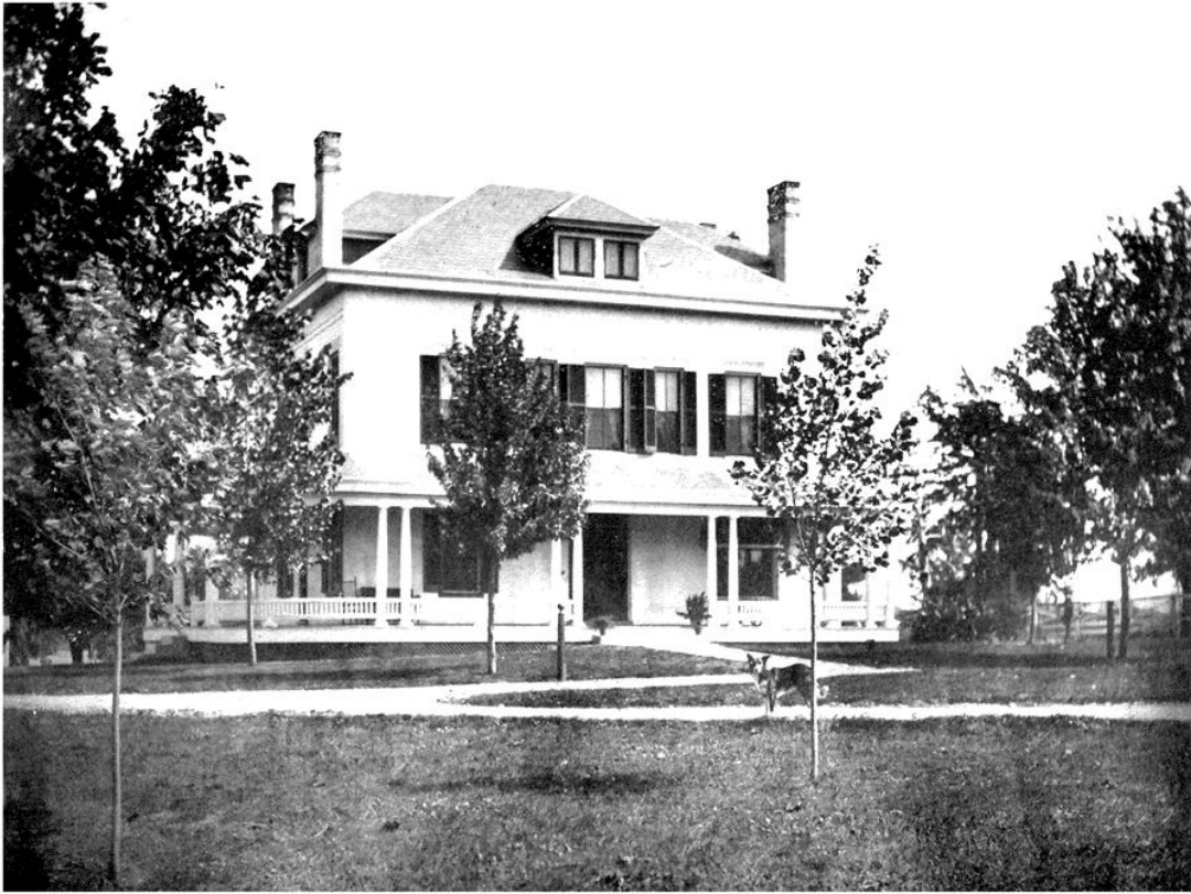
Front Elevation of Residence.
