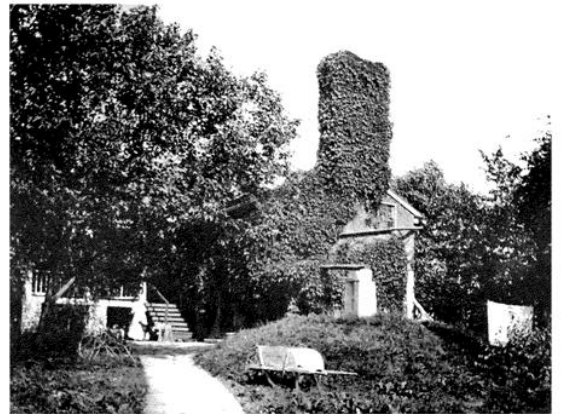
Rear View of Residence.
