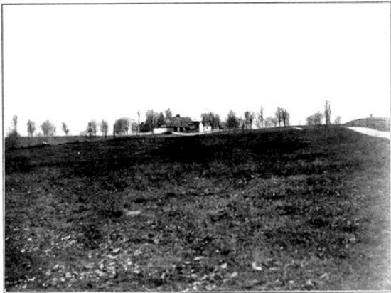
View of Century-old Barn.
