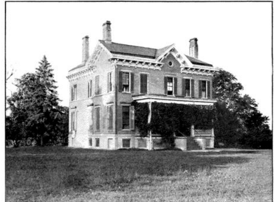
Rear View of Residence.
