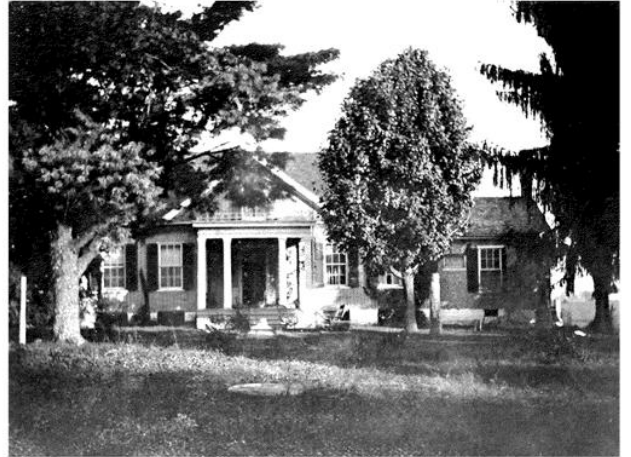
Cottage From the Roadway.
