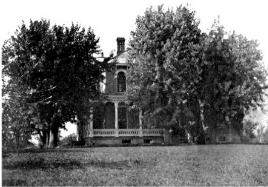
Front Elevation of Residence.
