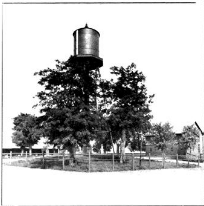
The Large Water Tower That Supplies the Farm With Water.
