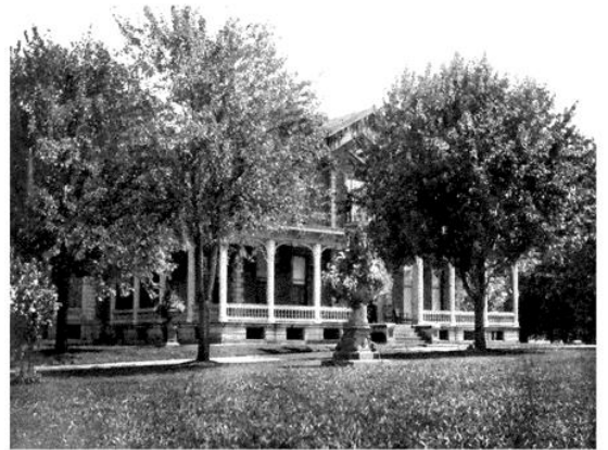
View From the Southwest.
