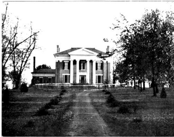
Front Elevation of Residence.
