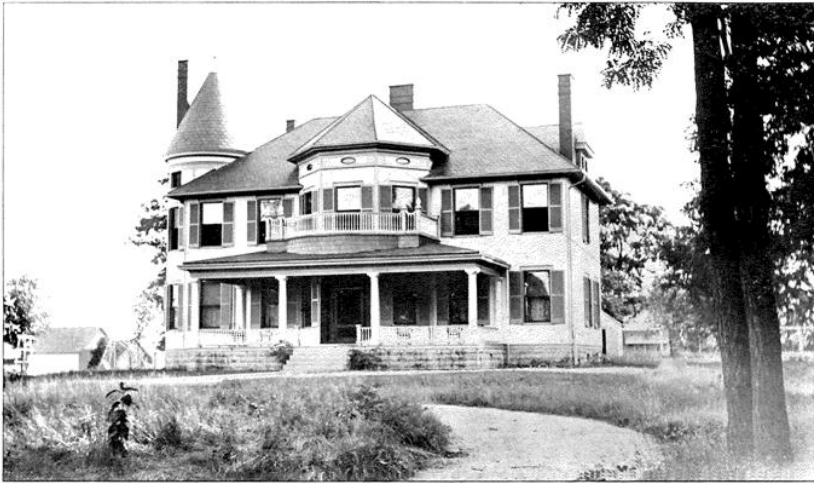
Front Elevation of Residence.
