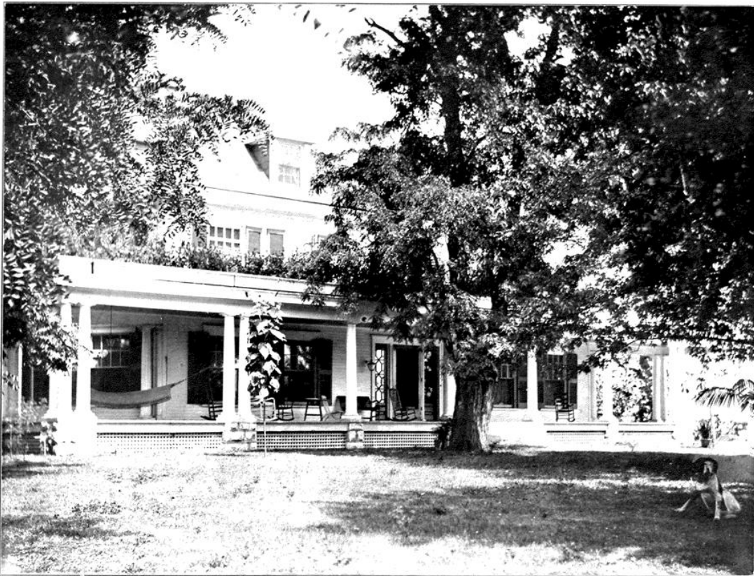
Front Elevation of Residence.
