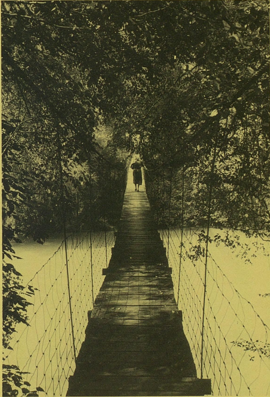
THE SWINGING BRIDGE AT WENDOVER
