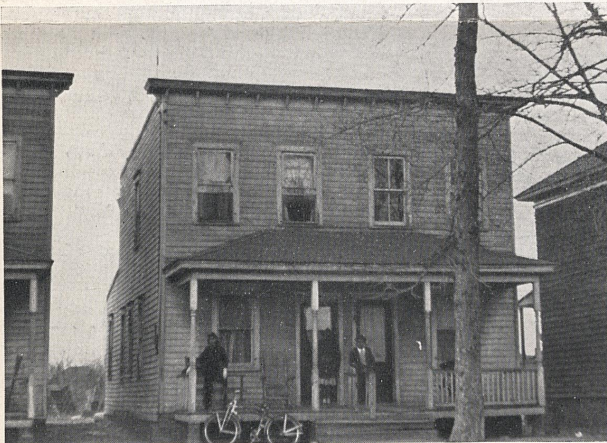
Street, tree, house, Garfield Court site, before demolition.
