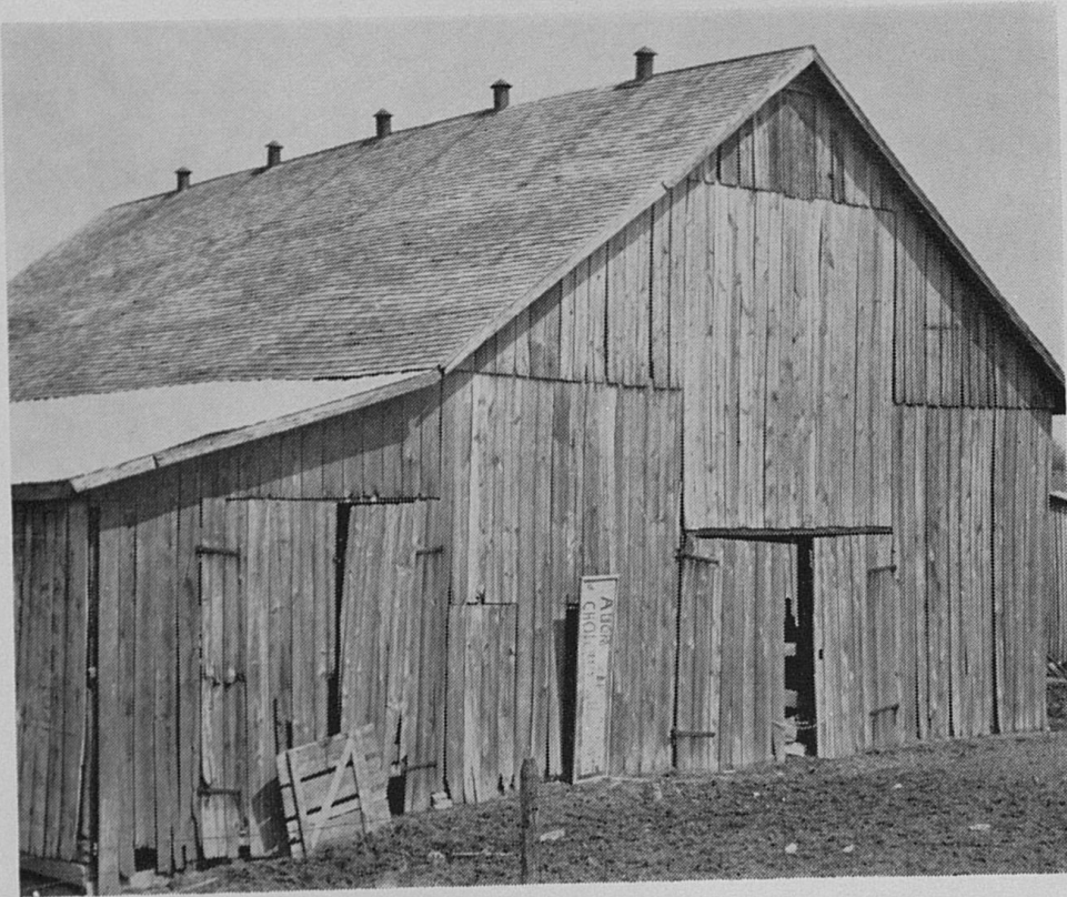
Fig. 3.— You have little control over curing conditions in a barn such as this. Sheds placed on the sides of a burley barn cut off ventilation completely. Also, ridge ventilators are useless.
