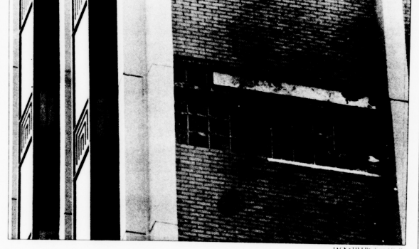
A large section of bricks on the extreme left side of the western face of Blanding Tower, the University's largest residence hall for women, was removed by Physical Plant Division workers yesterday with a crane. The brick tries that hold the outside brick panel to the inside brick wall came loose Tuesday and forced the eight-foot by 12-foot section of the South Campus residence hall to bulge outward, PPD officials said. Residents in rooms closest to the section were evacuated.
