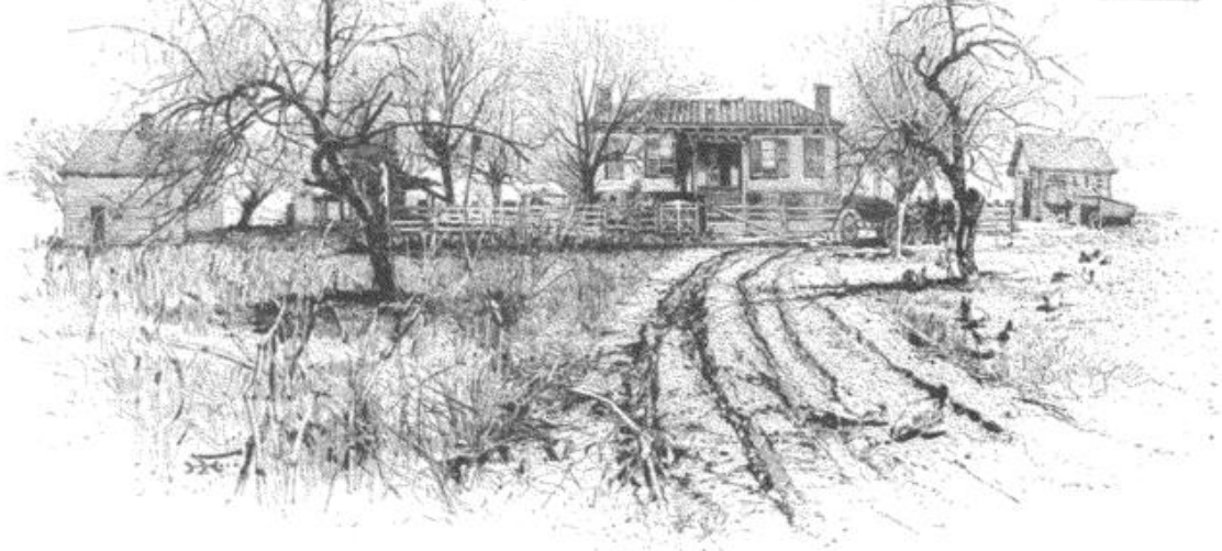
THE CREW HOUSE. THE UPPER PICTURE SHOWS THE OLD HOUSE, AND IS FROM A COLOR-SKETCH TAKEN SOON AFTER THE WAR; THE NEW HOUSE SHOWN IN THE LOWER PICTURE IS FROM A PHOTOGRAPH TAKEN EARLY IN 1885.
