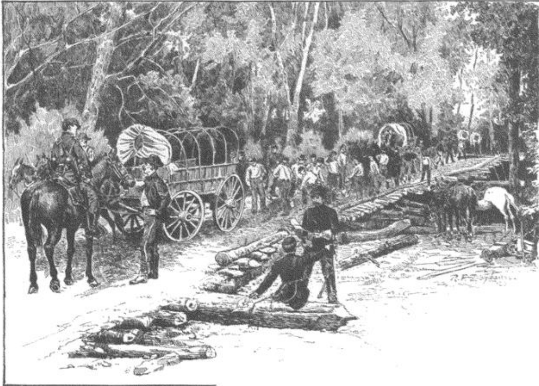
UNION TROOPS BUILDING THE CORDUROY APPROACHES TO GRAPEVINE BRIDGE. FROM A WAR-TIME PHOTOGRAPH. It was mainly by this bridge that the Union troops were withdrawn the night after the battle of Gaines's Mill.
