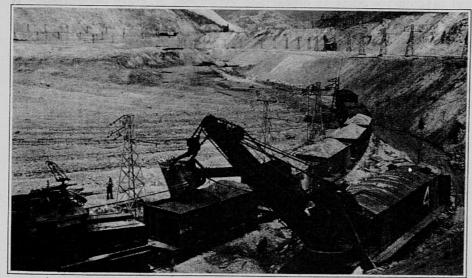
FIGURE 14.— A REMODELED SHOVEL LOADING ORE AT AN OPEN—CUT COPPER MINE
