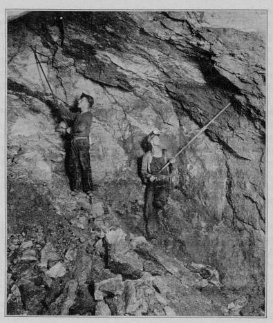
FIGURE 45.— BARRING DOWN LOOSE ROCKS IN UNDERGROUND WORKING PLACES
