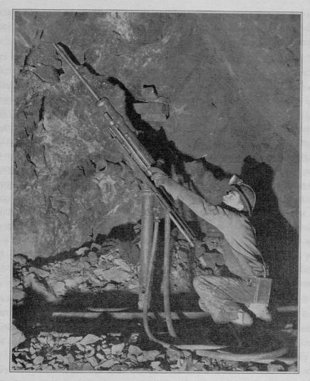
FIGURE 34.- AN IMPORTANT STEP IN METAL PRODUCTION IS THE BREAKING OF ORE BY DRILLING AND BLASTING
