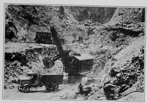
FIGURE 17.— TRUCK HAULAGE IN AN OPEN—CUT COPPER MINE
