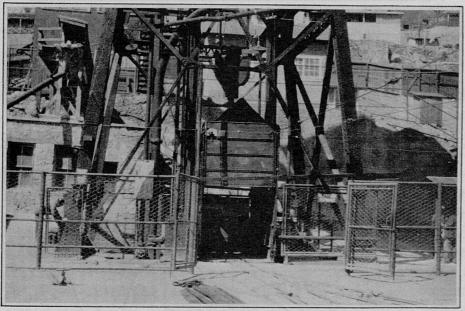
FIGURE 20.- ORE, MEN, AND MATERIALS MOVE THROUGH THE SHAFT AT AN UNDERGROUND MINE
