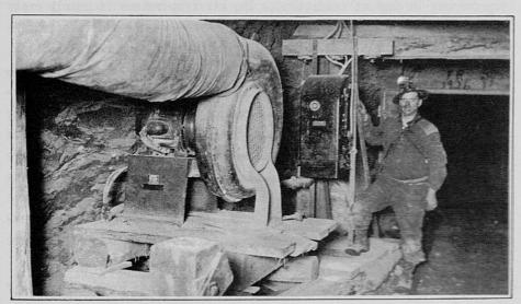
FIGURE 40.— INCREASED USE OF MECHANICAL VENTILATION DEVICES WAS NECESSARY WITH THE EXPANSION OF OPERATIONS AT UNDERGROUND MINES
