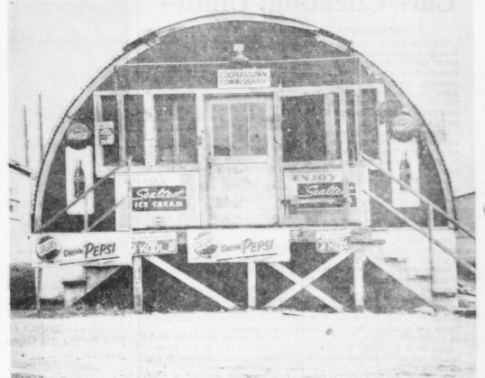
COOPERSTOWN COMMISSARY —A "colorful," modern, fully equipped store, is counted as one of UK's assets. Behind this building, to the left, is the Cooperstown laundry, about one fourth its size. The laundry has two sinks, a washing machine, a dryer, and an open drain in the floor for the rinsing basins.
