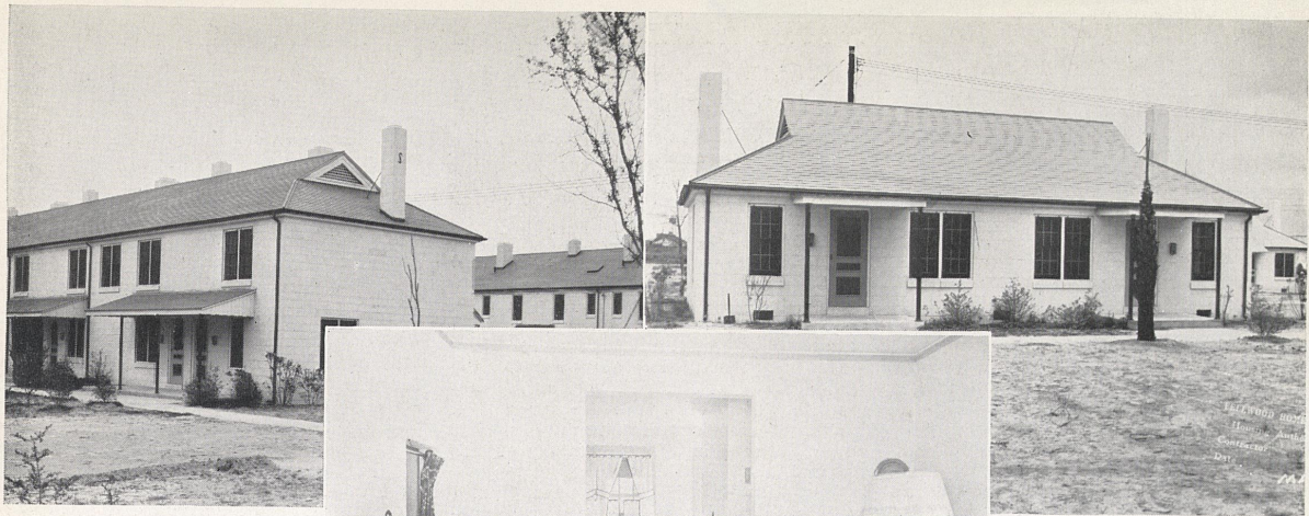
ABOVE.—Two views of Fellwood Homes in Savannah. The project is composed of 1-story twin houses and 2-story row houses. The concrete block construction is inexpensive, durable, attractive.
