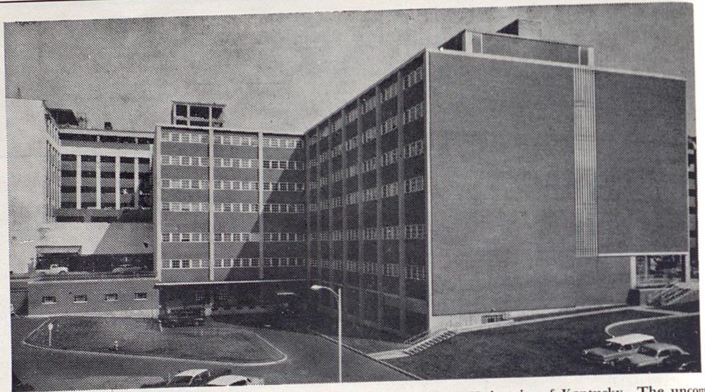
The new six-story, air-conditioned Medical Science Building at the University of Kentucky. The uncompleted portion at the left will be the 500-bed hospital.
