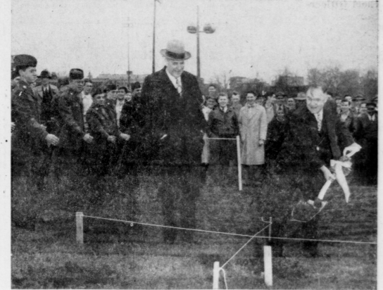
FIELDHOUSE GROUND BROKEN —Dr. Herman L. Donovan dug the first spadeful of dirt as excavation for the new $1,000,000 memorial field house began in April. Governor Simon Willis looks on.
