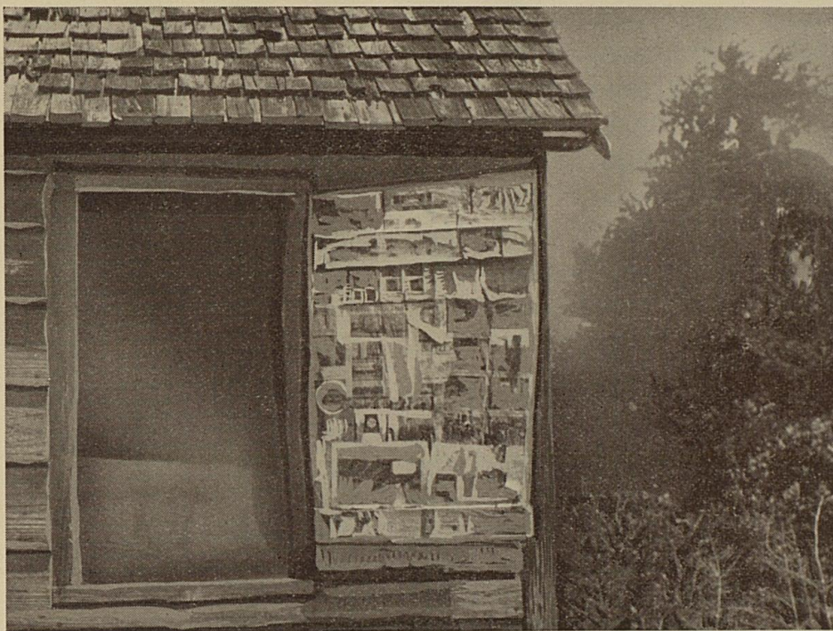
Close-up of open wooden shutter of Negro cabin on St. Helena Island, showing a frequent use of newspapers as papering material.
