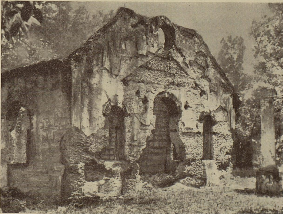
Ruins of White Church, St. Helena Island, Chapel of Ease to St. Helena's Episcopal Church, Beaufort, S. C. The construction is of tabby (a mixture of oyster shell and lime); built prior to the Revolutionary War; date unknown. Destroyed by forest fire.
