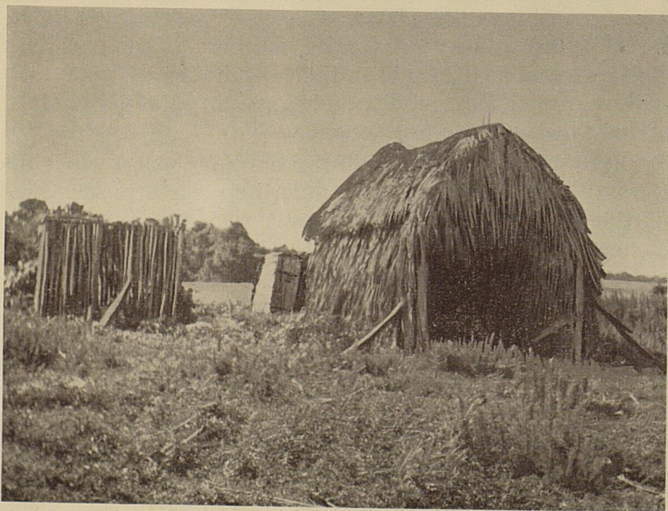
CRITTER HOUSE, made of palmetto fronds, a type of stable used to house domestic animals on St. Helena Island.
