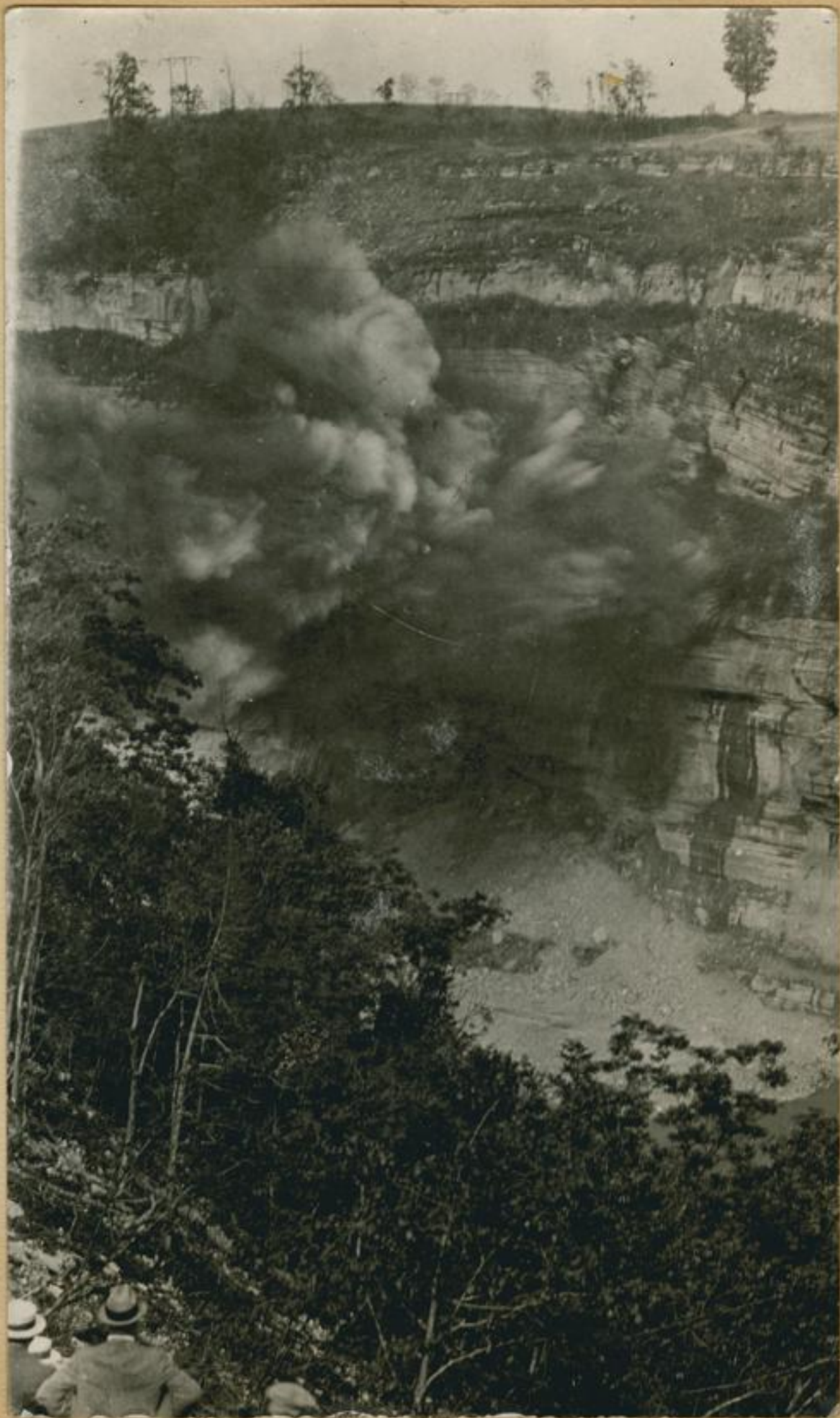
Big Blast at Dam - 40000 lbs of explosives
