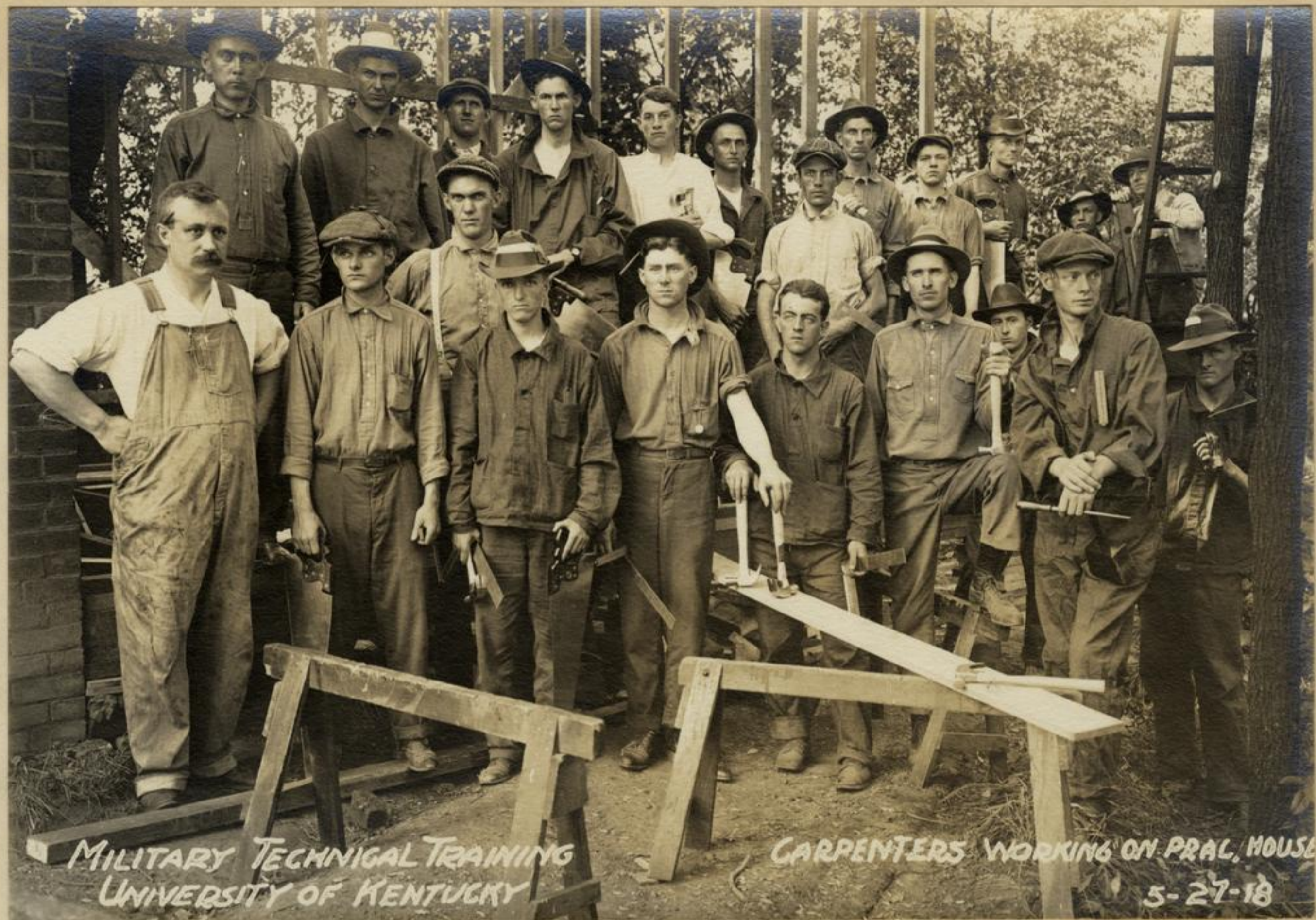
A Carpenter Section Before The Building Being Erected to be Used in the Training of Electricians in House Wiring Lexington, Kentucky
