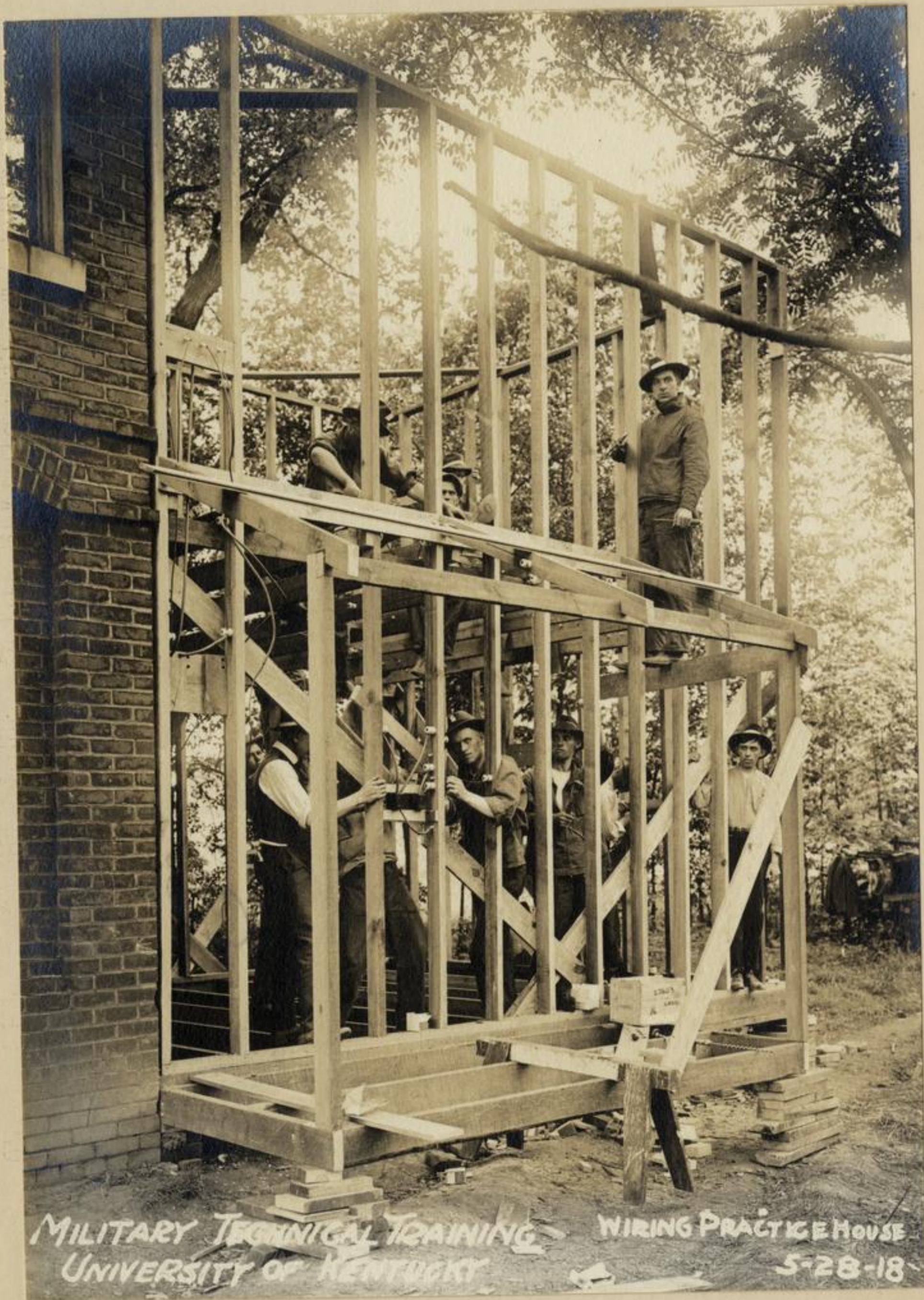
A Section of Electricians Doing House Wiring in the Building Especially Erected for their Training Lexington, Kentucky
