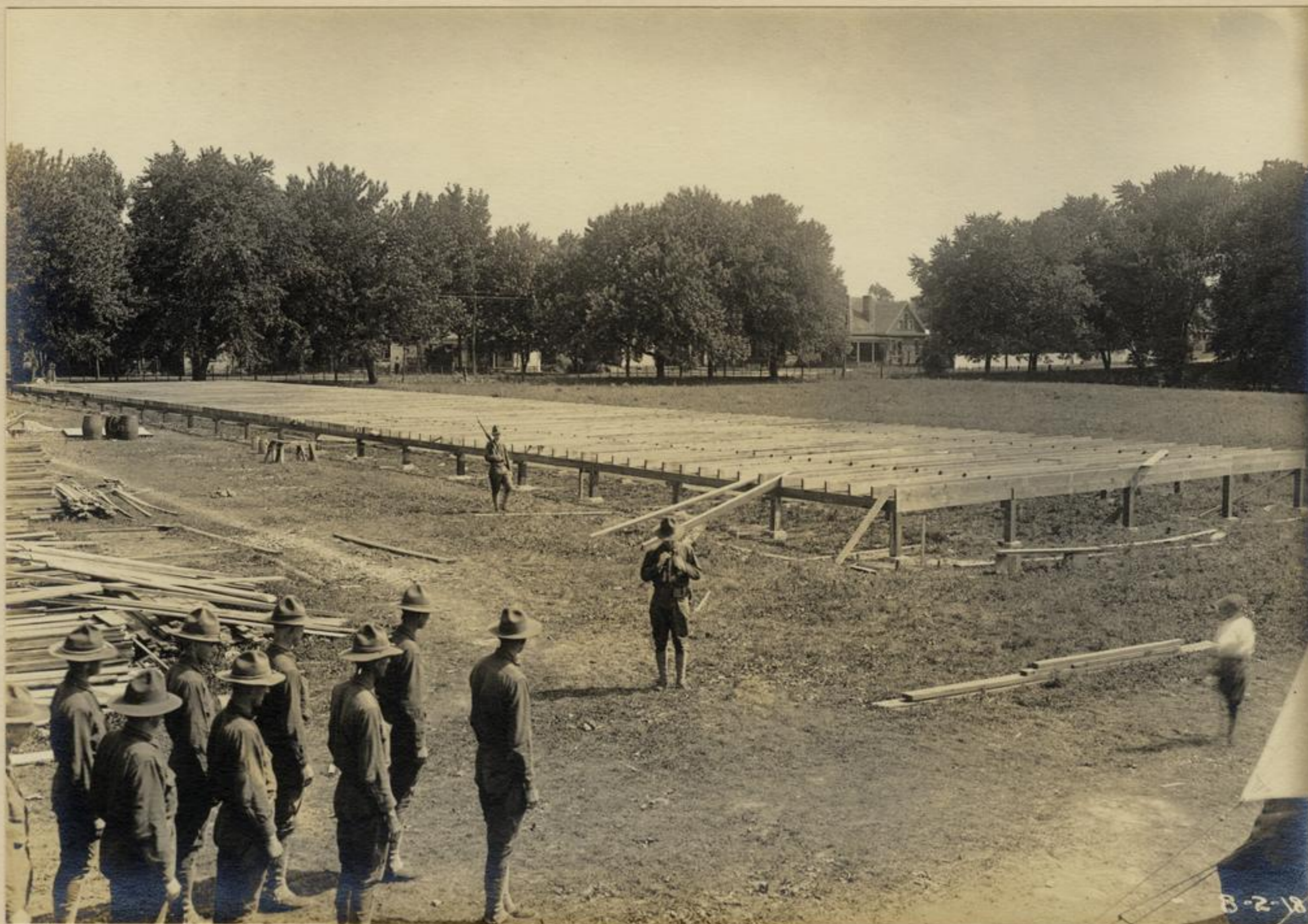
Showing Progress on Second Barracks
