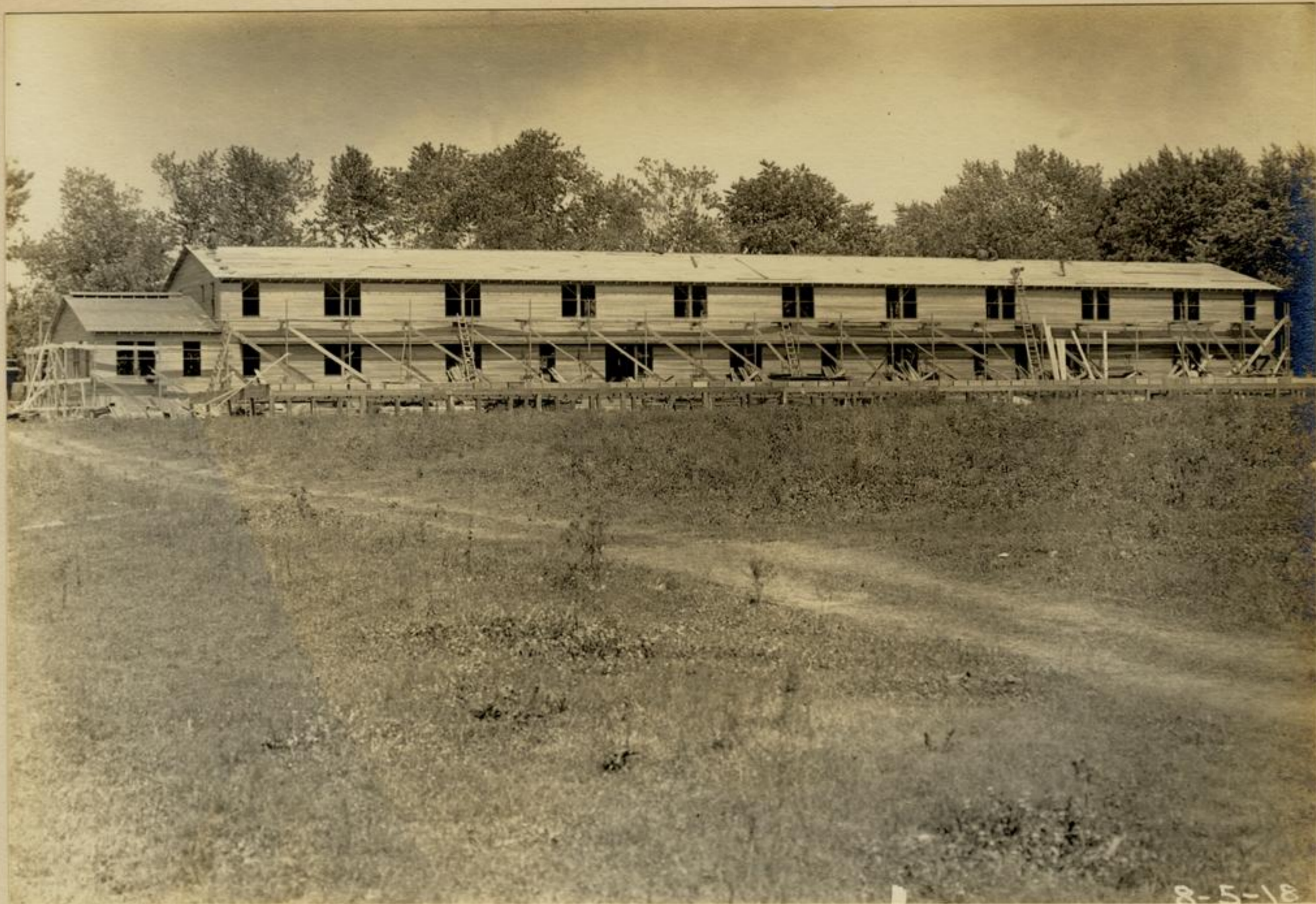
Showing Progress on First Barracks
