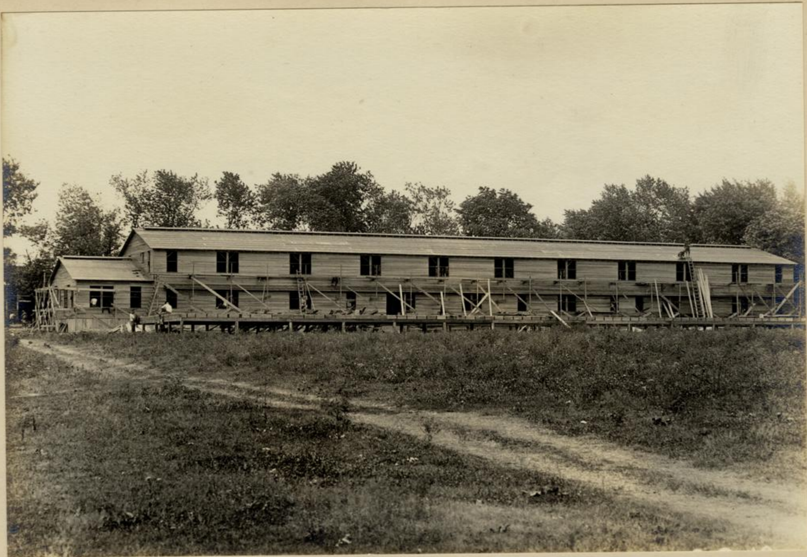
Progress on First Barracks
