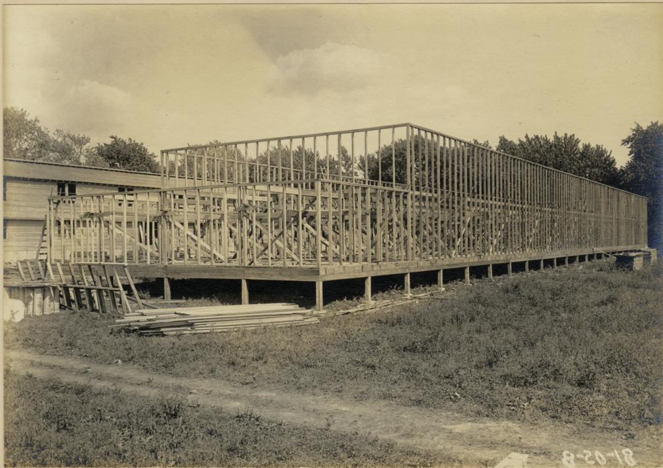
Showing Progress on Second Barracks
