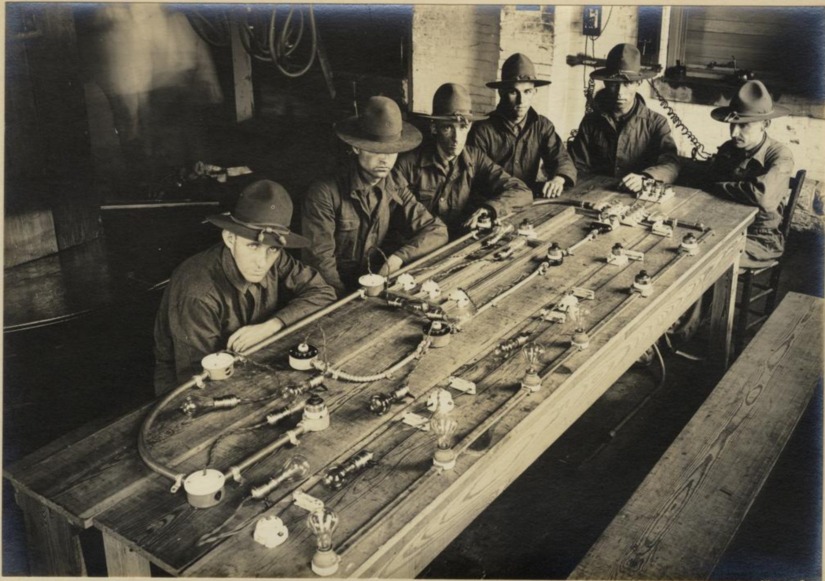
Electricians at Work on Wiring Problem
