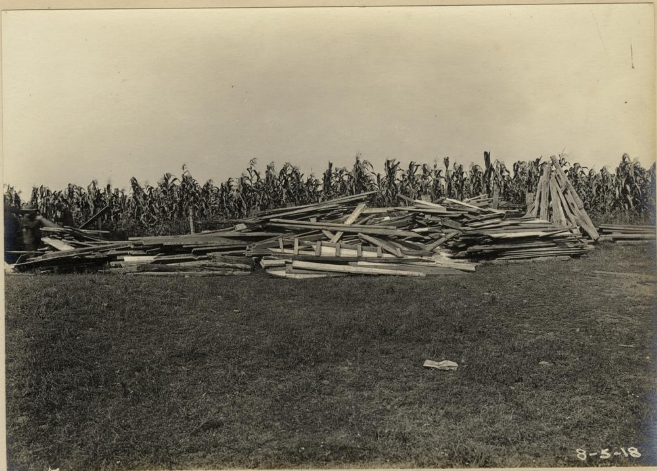
Converting an Old Lumber Pile Into a Substantial Structure by Some Men of the Carpenter Section
