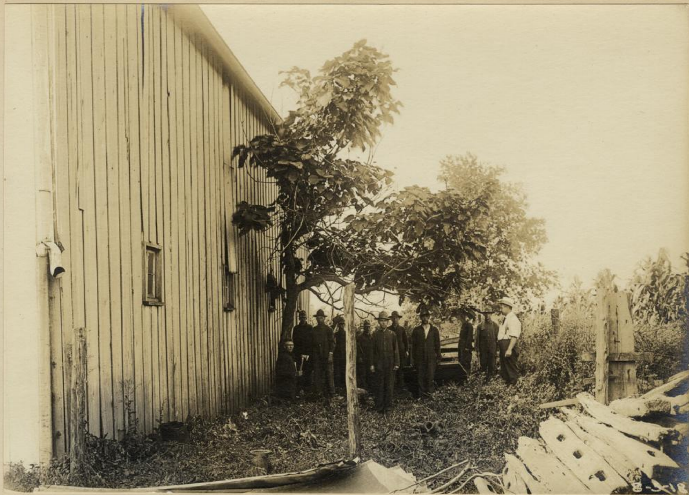
Converting an Old Lumber Pile Into a Substantial Structure by Some Men of the Carpenter Section
