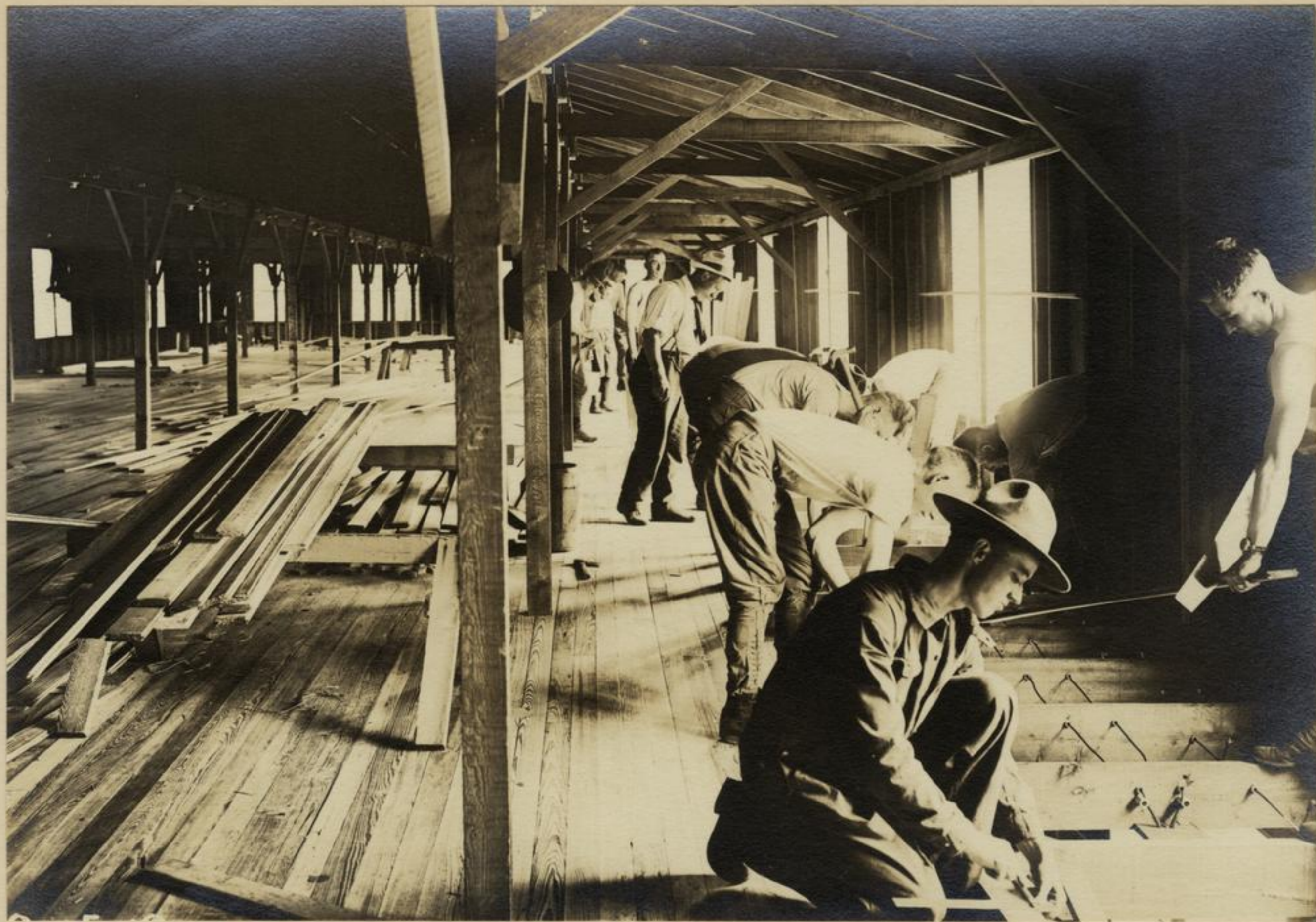
Carpenters at Work
