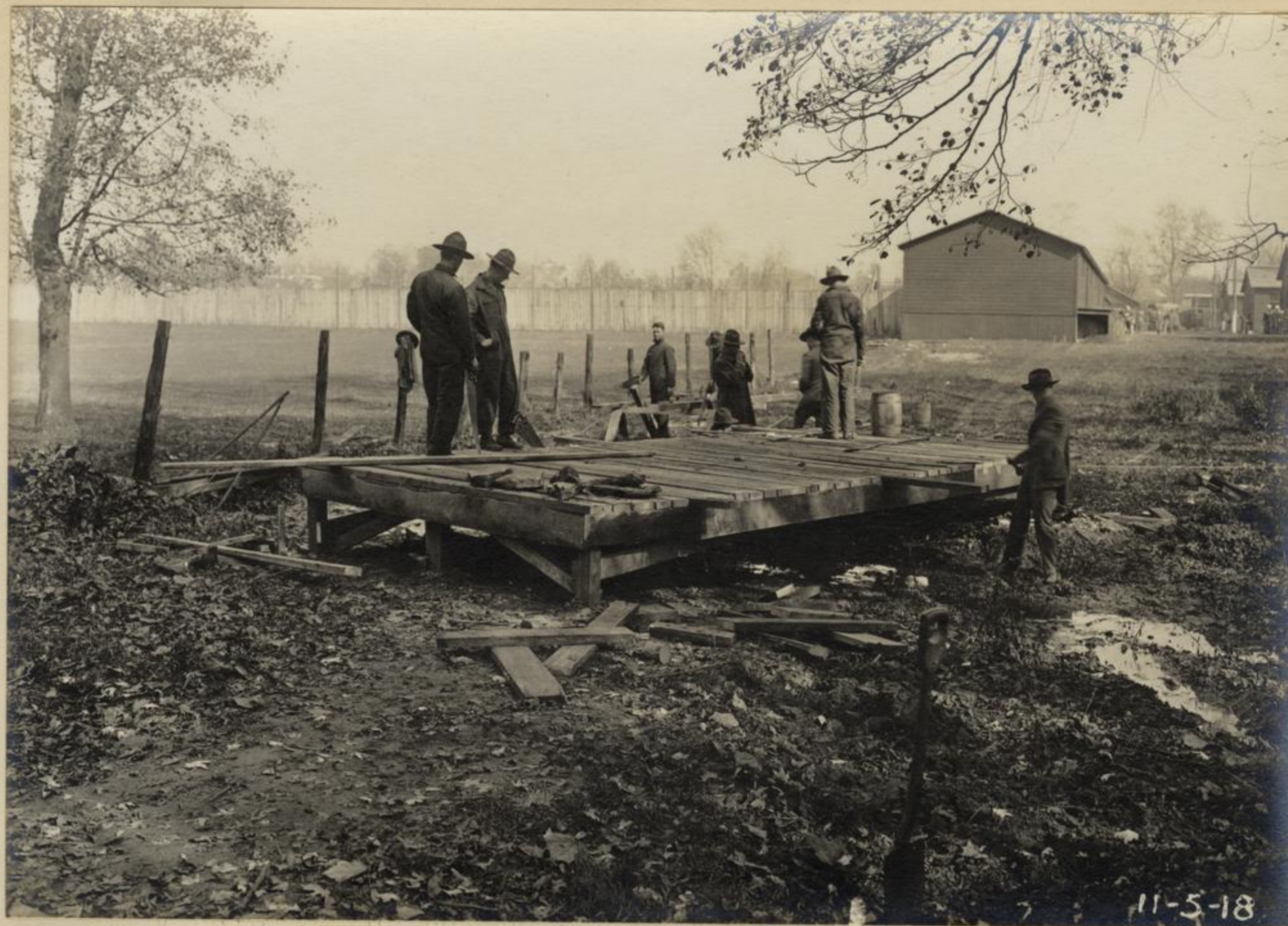
An exercise in bridge building by the carpenters, Section B.
