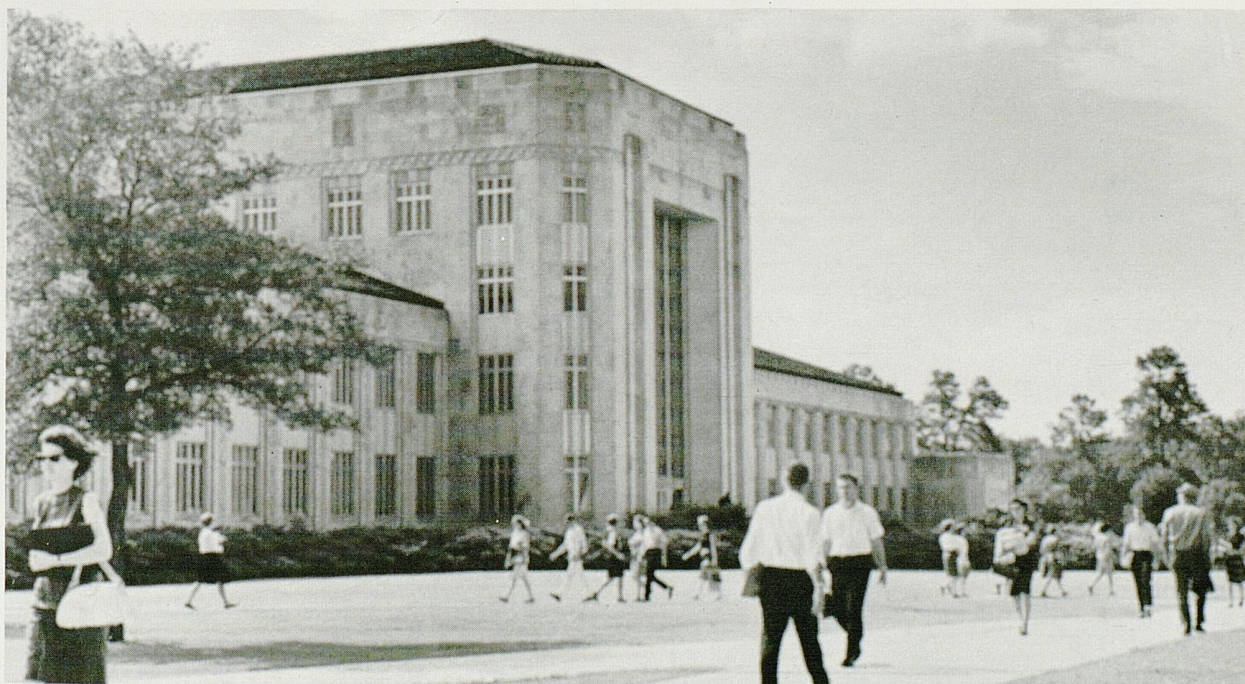
EZEKIEL W. CULLEN BUILDING - ADMINISTRATION BUILDING
