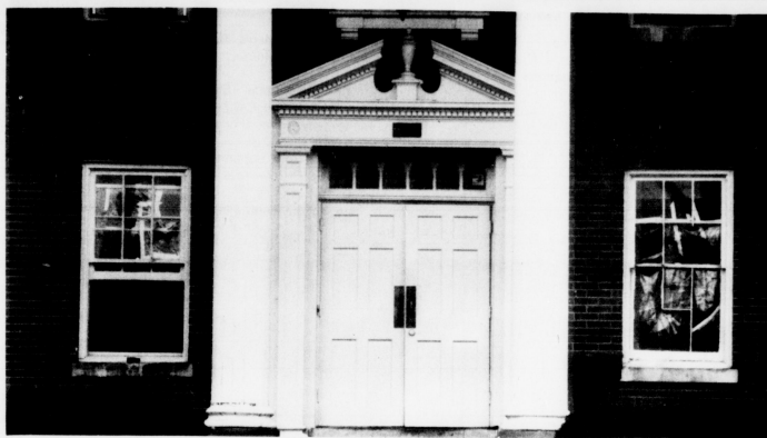
Six windows of the Delta Tau Delta fraternity house, located at 1410 Audubon Ave., were smashed out early
