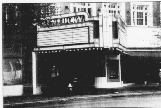
The Kentucky Theatre, which was closed after a 1987 fire, finally will reopen in April. Vice Mayor Pam Miller, who pushed for renovations of the movie house, said it will keep its traditional format.
