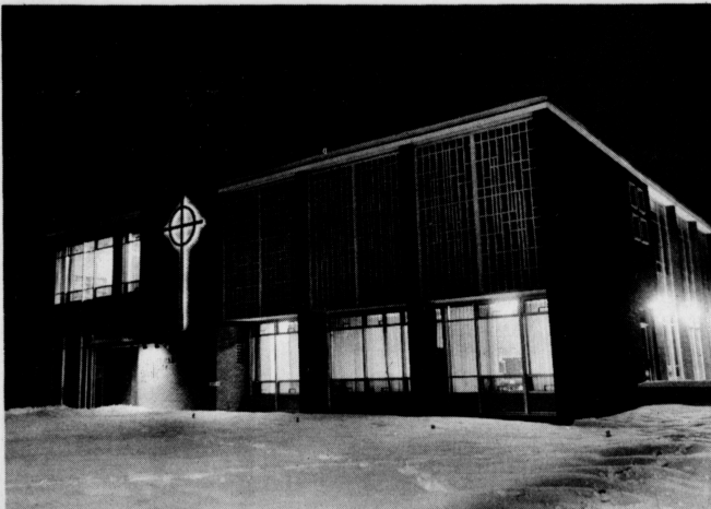
The Presbyterian Student Center, Located On Rose Street.
