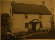
THE GEORGE BOOSE HOUSE, NEAR LEBI KILN, PENNSYLVANIA
