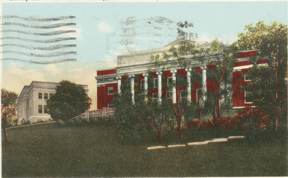
Library and Administration Buildings, Western Kentucky State Teachers' College, Bowling Green, Ky.
