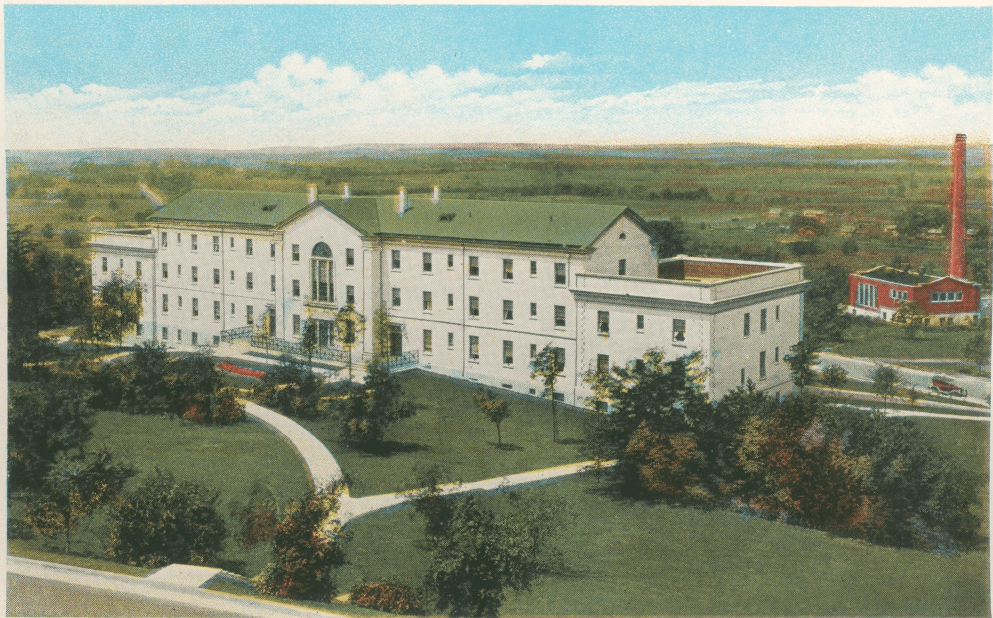
WEST HALL AND HEATING PLANT
