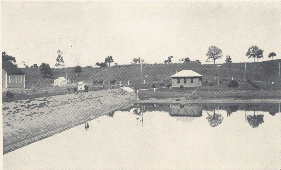
PUMP HOUSE AND DAM, CARLISLE WATER WORKS, CARLISLE, KY.
